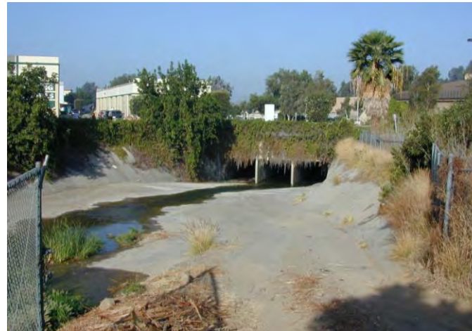
Concrete or other man made materials should not be used to stabilize channel banks
