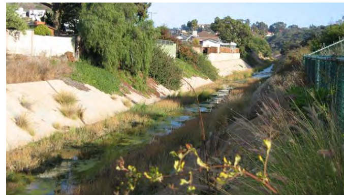
Hard surfaced channels such as Tecolote Creek increase velocity, prevent groundwater recharge and offer little wildlife habitat
