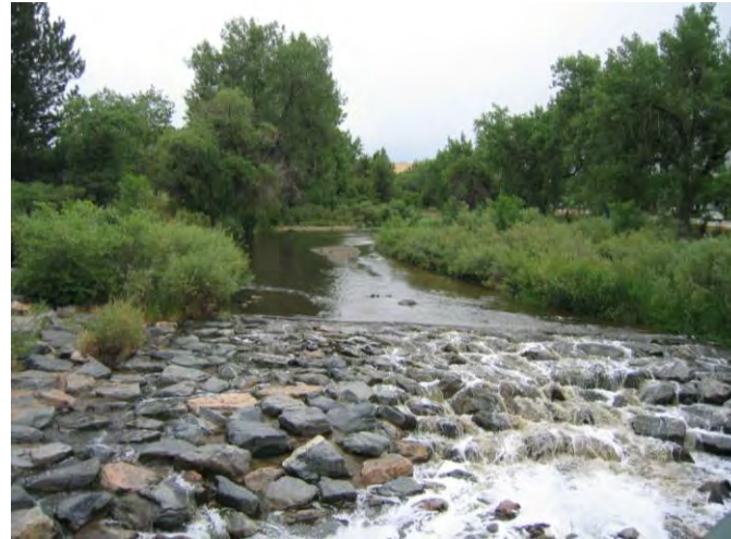
Example of natural stone used to dissipate flows and allow for wildlife movement
