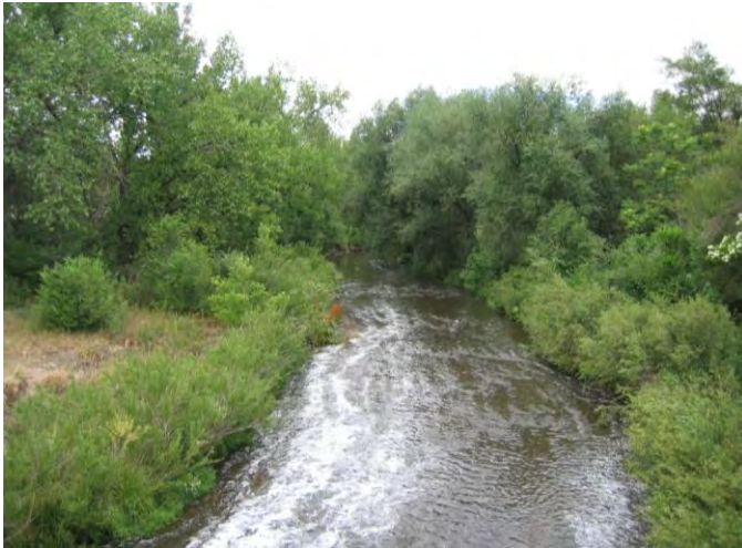
Rehabilitated Platte River in Colorado designed to be natural in appearance by utilizing native materials and gentle slopes
