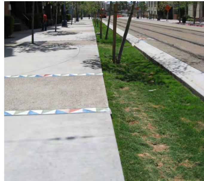
Example of an infiltration basin
