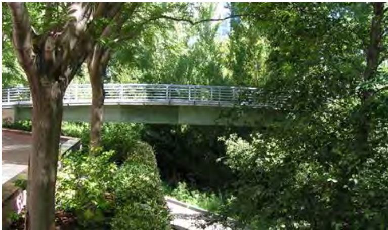
Example of a bridge complimenting the river park
