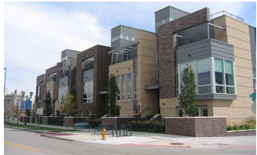
Example of varying building form, massing and façade treatment
