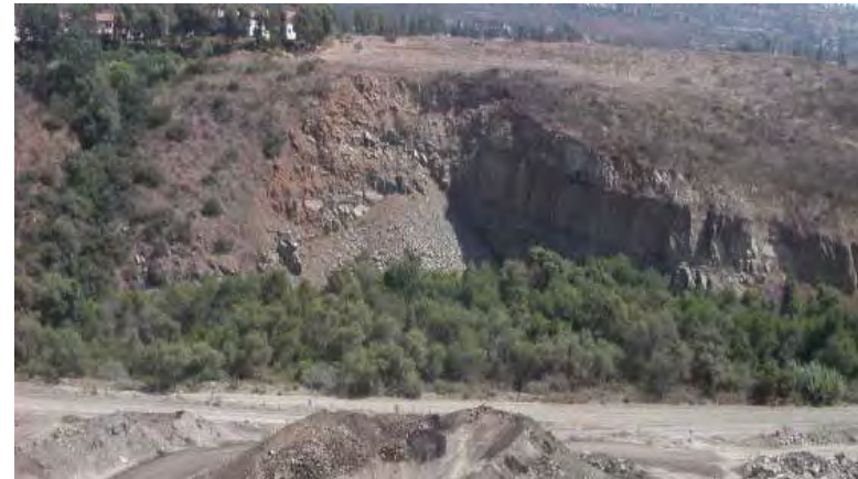
The reclamation and development of Superior Mine is a significant opportunity to improve the condition of the River and wildlife habitat
