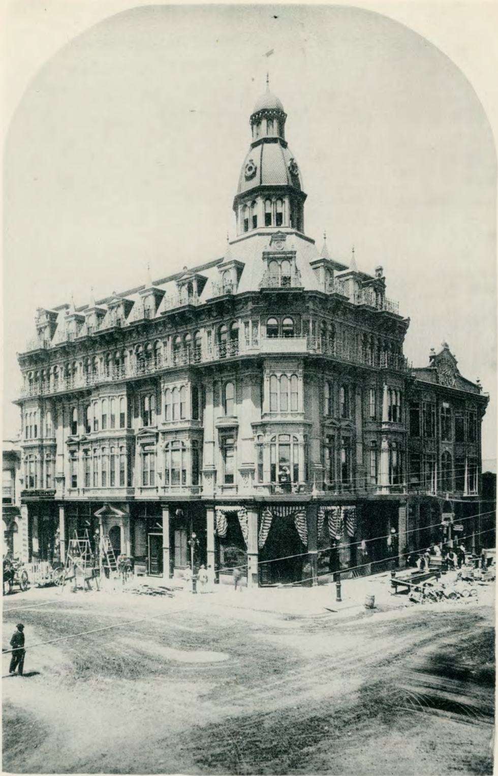
Morse-Pierce Building, corner Sixth and F streets, San Diego.
