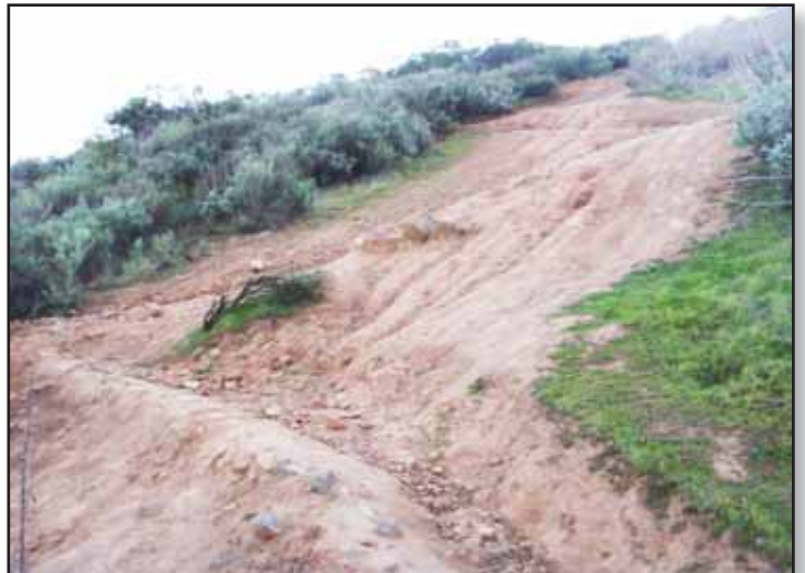
One of many sections along the Kwaay Paay trail that is excessively steep and eroding that is recommended for reroute (MG-R9)
