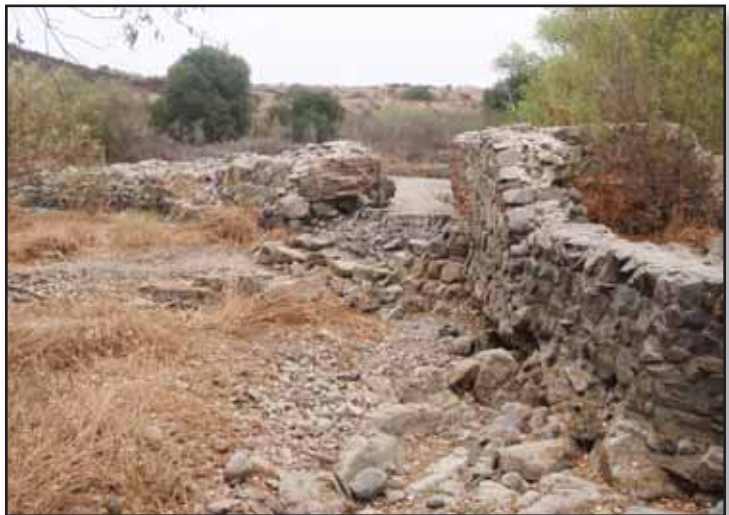
Old Mission Dam with no flowing water (fall 2013)
