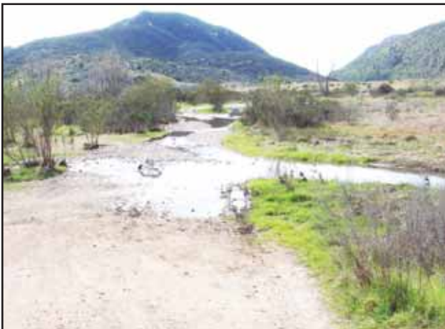
Park road recommended for closure (FM-R39)
