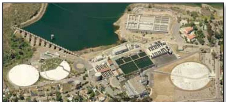
Alvarado Water Treatment Plant (Source Bing 2012)
