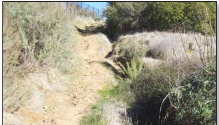
Eroding section of Shepherd Canyon trail recommended for local reroute (FM-R21)
