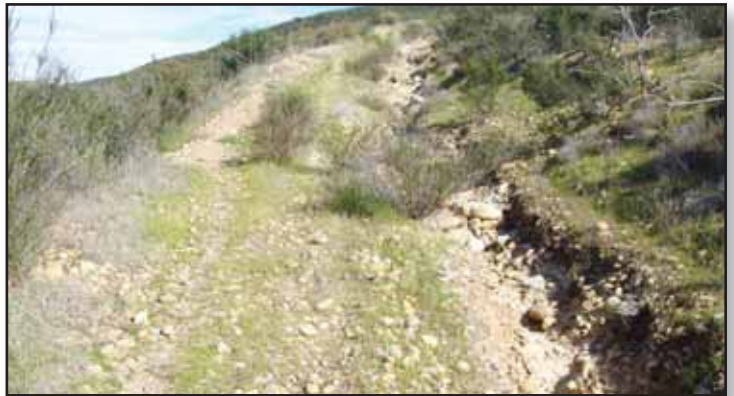
Section of old road cut recommended for closure and replacement (EE-R4)
