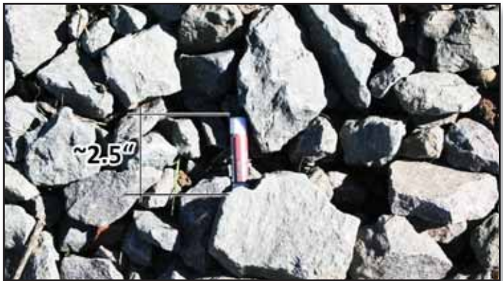
Utility road surfaced with 2-6 inch rock that is difficult to walk or ride on and unsafe to run on
