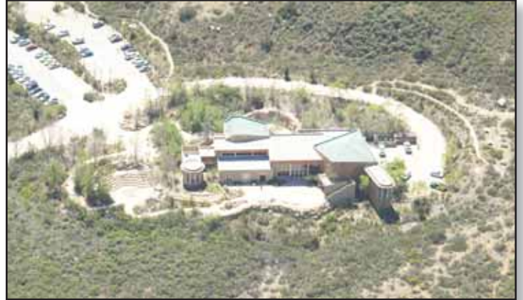
Native coastal sage scrub adjacent to the Visitor and Interpretive Center requiring periodic brush management activities
