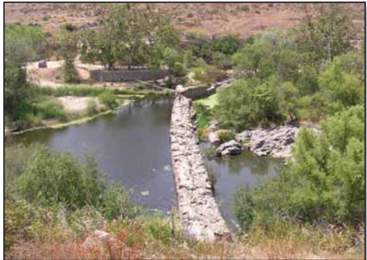
Post-Dredging at Old Mission Dam (Oct 2007)
