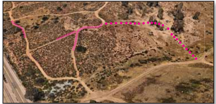
A section of old ranch road to be assessed for localized improvements to address steepness and erosion concerns (EE-R36) and several sections of old ranch road recommended for closure (EE-R35)
