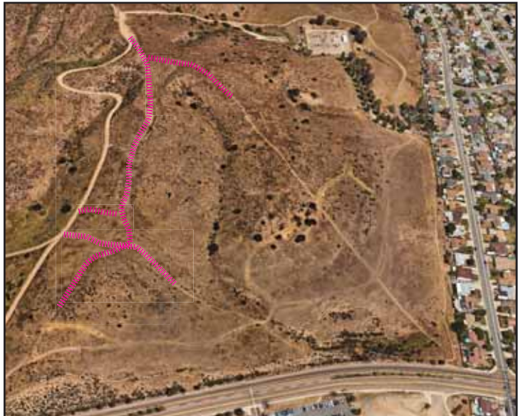
Sections of old ranch road recommended for closure (EE-R33,34)
