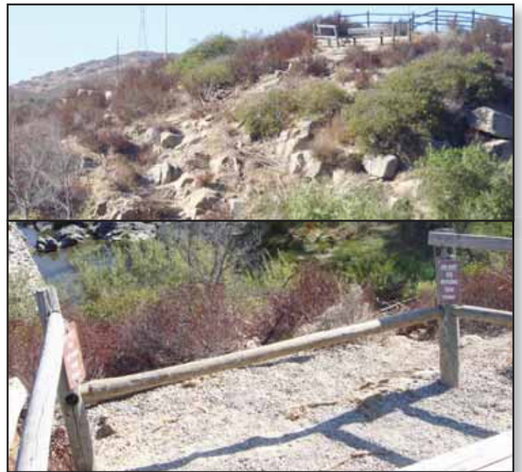
The Old Mission Dam overlook needs to be reconstructed and the slope below revegetated to discourage off trail use (FM-F3)
