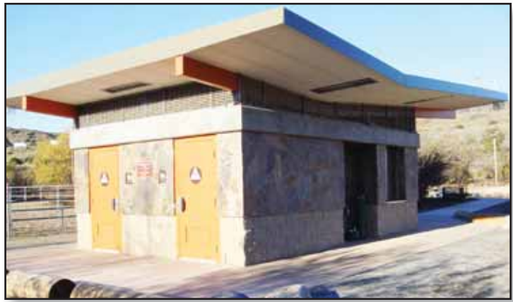
New comfort station at the East Fortuna Staging area
