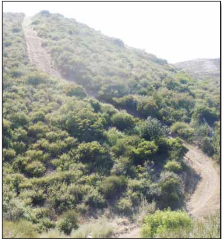
Existing utility access road with greater than 70% slope
