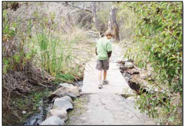
Drainage requiring improved bridge crossing or trail reroute as part of the San Diego River Trail improvements (MG-R2)
