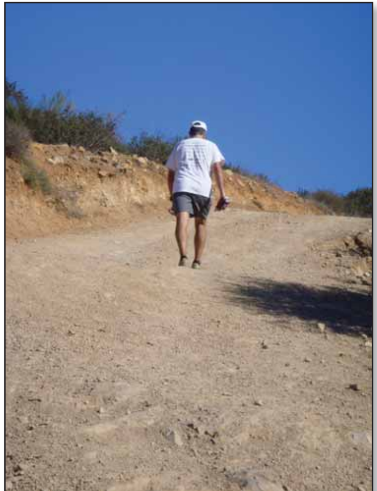
Example of Utility Access Road that is extremely steep making recreational use difficult
