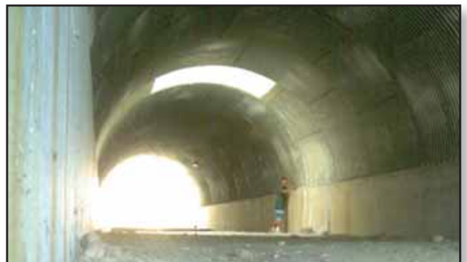
Surveillance camera within wildlife tunnel being stolen (FM-H1)
