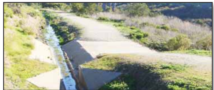
Urban runoff diversion channel (LM-M6)
