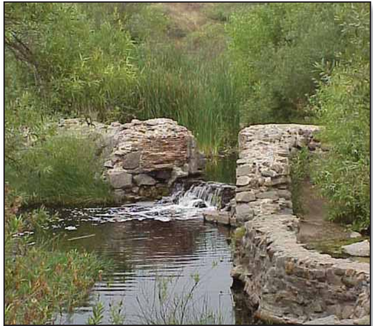
Old Mission Dam with water flowing over the sill
