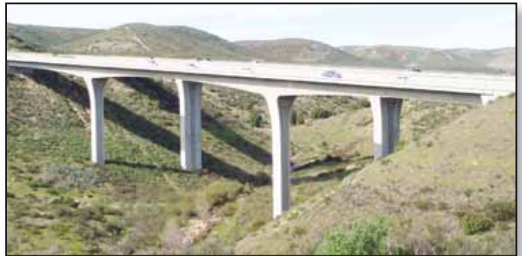
SR-52 undercrossing into Oak Canyon
