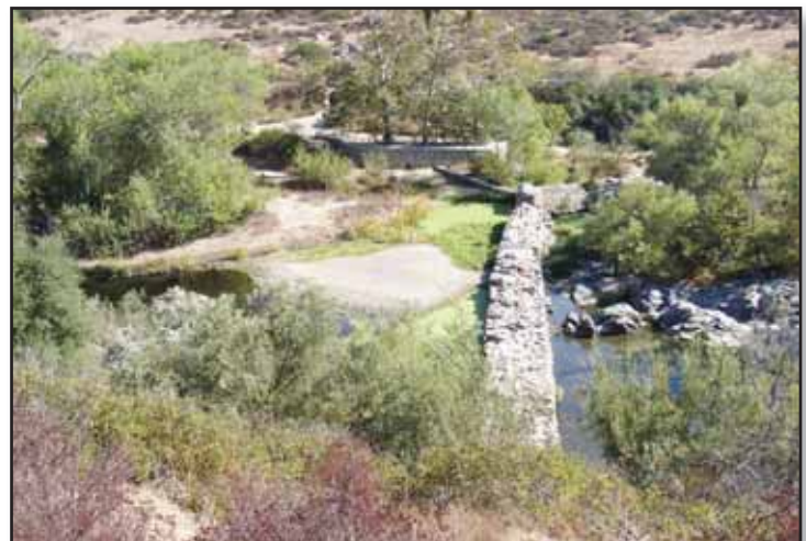
Post-Dredging at Old Mission Dam showing new sediment accumulation ( 2012)
