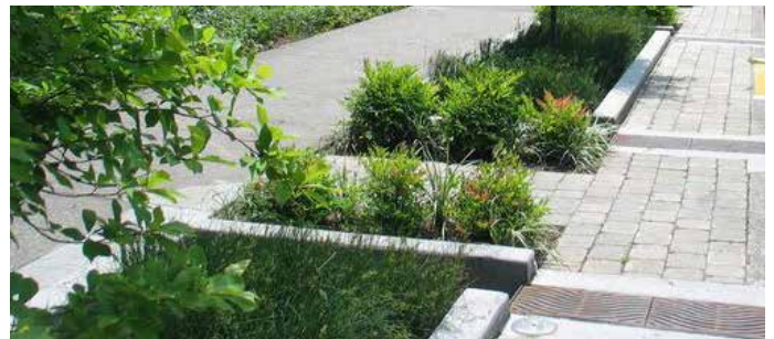
Green infrastructure can help filter storm water before it enters the conveyance system.
