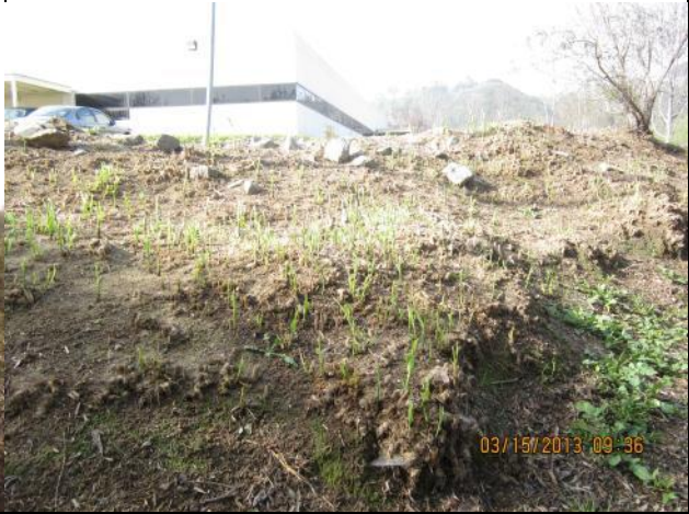
PHOTO 4 NOTES: Staging area.
