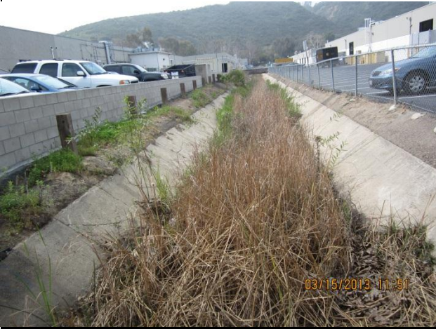
PHOTO 3 NOTES: From culverted facing southwest.
