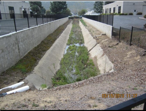
PHOTO 1 NOTES: Northeast end facing southwest (upstream).
