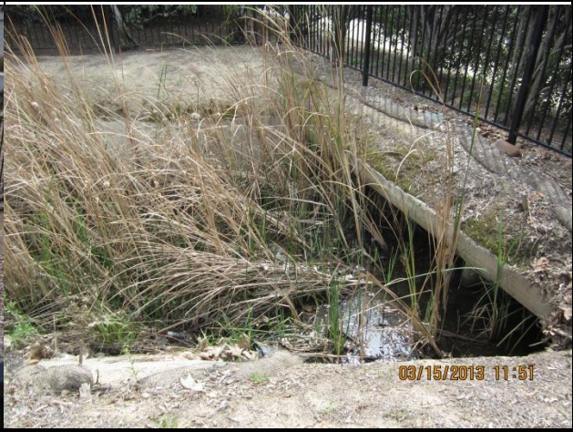
PHOTO 2 NOTES: Culverted road crossing.
