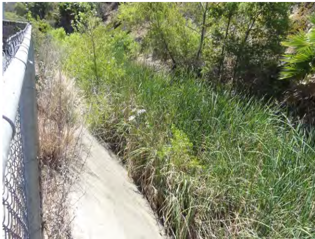
From North side of channel in Reach 2, looking upstream
