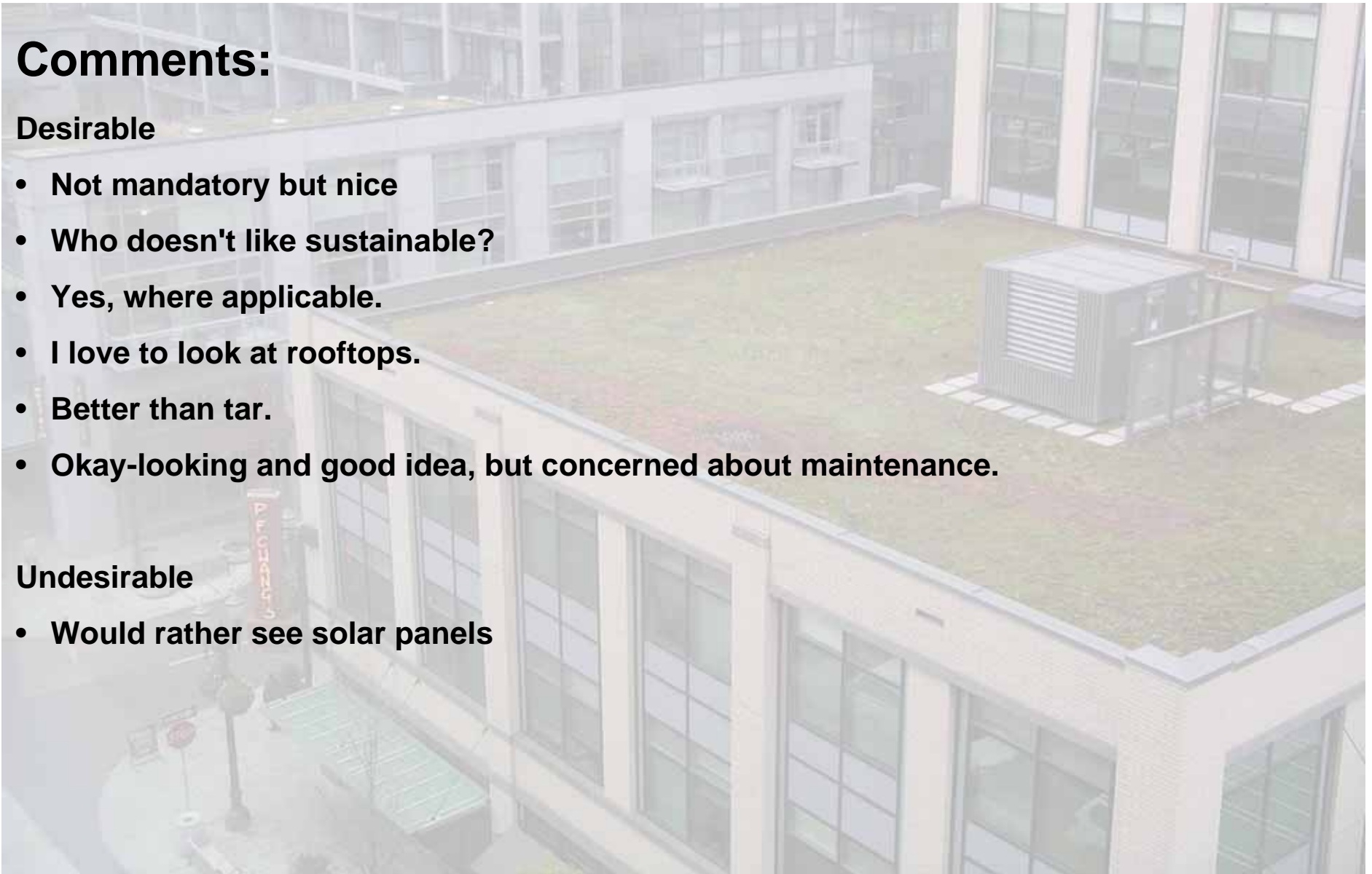
green roof on commercial building
