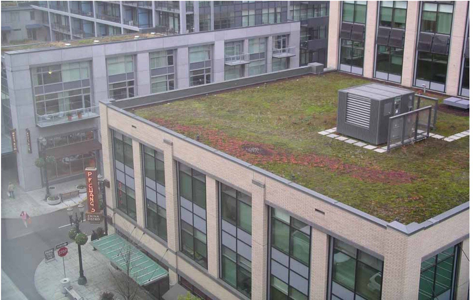
green roof on commercial building
