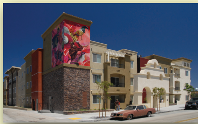
La Entrada Family Apartments Barrio Logan
