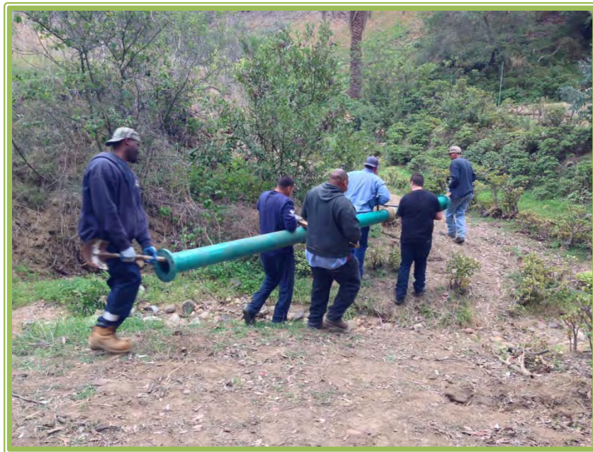
Spruce Canyon Pipe Repair
