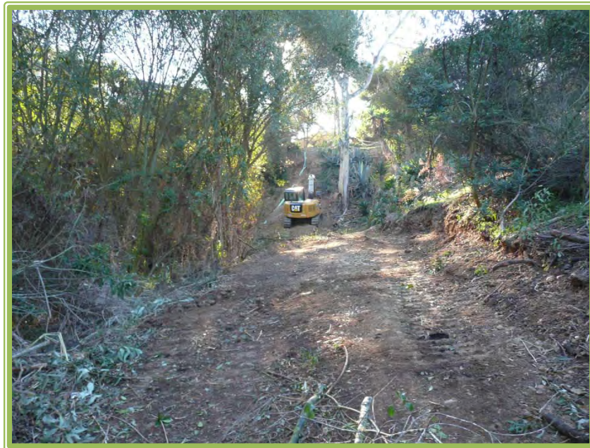
Buchanan Emergency Sewer Blockage Emergency Access and Repair
