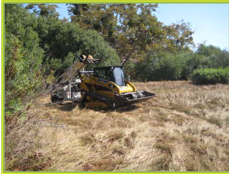
Lopez Canyon –Towing Cleaning Equipment to Manhole 13
