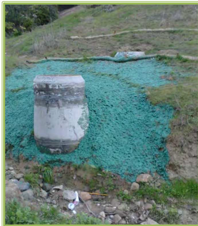
Spruce MH 220 Replacement Revegetation (erosion control) Project
