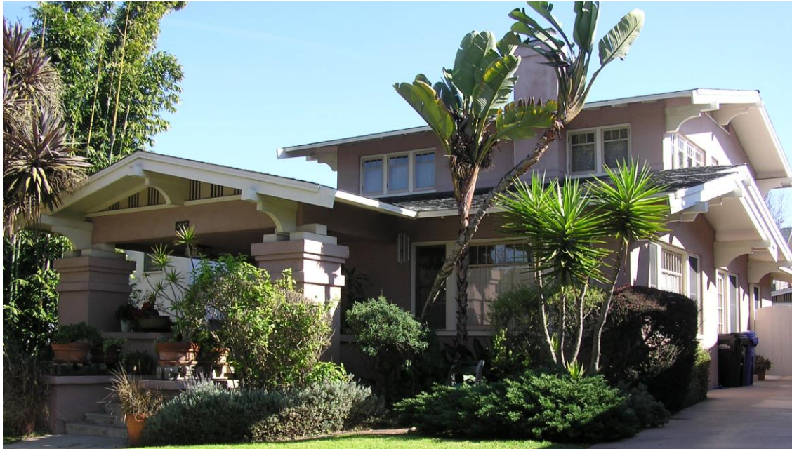
Dyar and Grace Hazelrigg House, 4247 Arden Way, Resource #495 Photos courtesy of Katherine Hon, December 31, 2008
