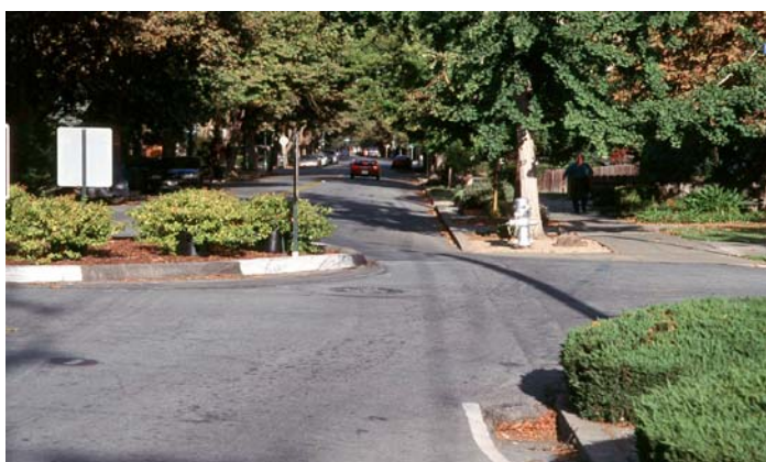
Below: Example of a temporary roundabout. Shrubs are in temporary planters.
