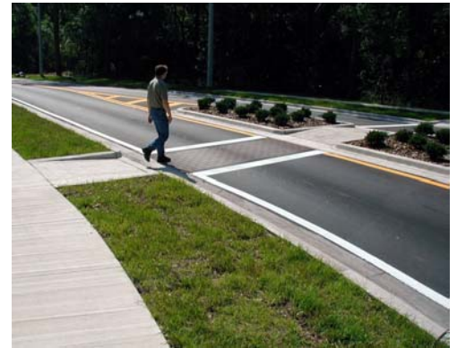
The Colima Street roundabout will be a similar size and shape as those illustrated above
