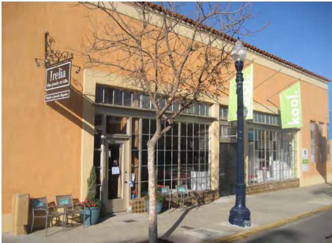
Adaptive reuse will ensure that historic character and scale is maintained as the neighborhood evolves.
