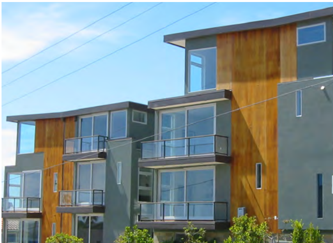
Materials should be selected that complement and respond to San Diego's climate and maximize views and natural light and ventilation.
