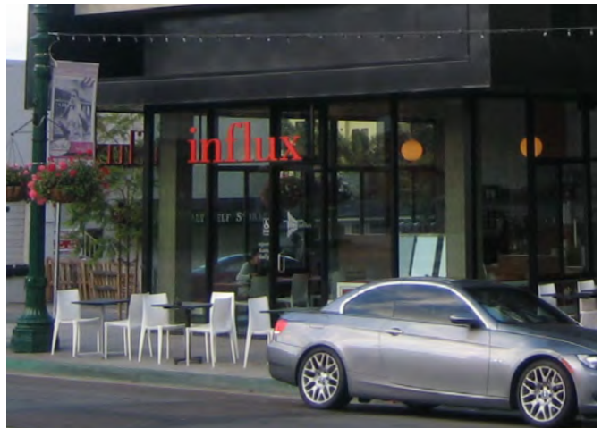
Signs should be integrated with overall building design with a simple and clear message.
