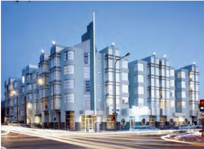
Lighting of buildings should be intergrated into the building design and employ fixtures that reflect overall design approach.
