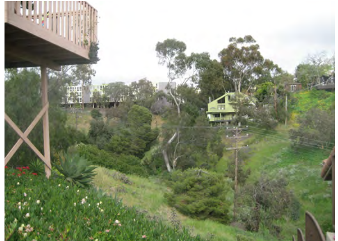
Structural supports for buildings along the canyon interface should be minimal in profile.
