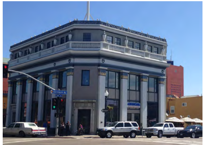
The adaptive reuse of historic buildings for commercial purposes is highly encouraged.
