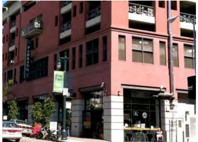
Parking garages, if necessary, should be lined with commercial or residential units and screened on upper stories to reduce perception of parking.
