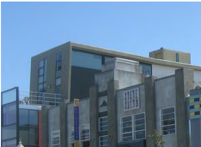
Mechanical penthouses and rooftop equipment should be setback from the primary building façade and screened.
