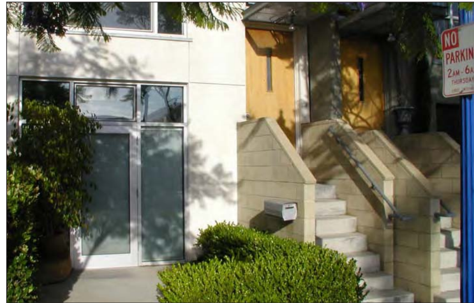
Live / Work Building Entry
