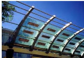
Example of Art as Part of a Building's Structure
