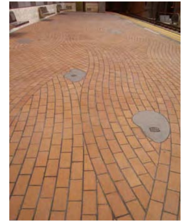
Example of Enhanced Paving
