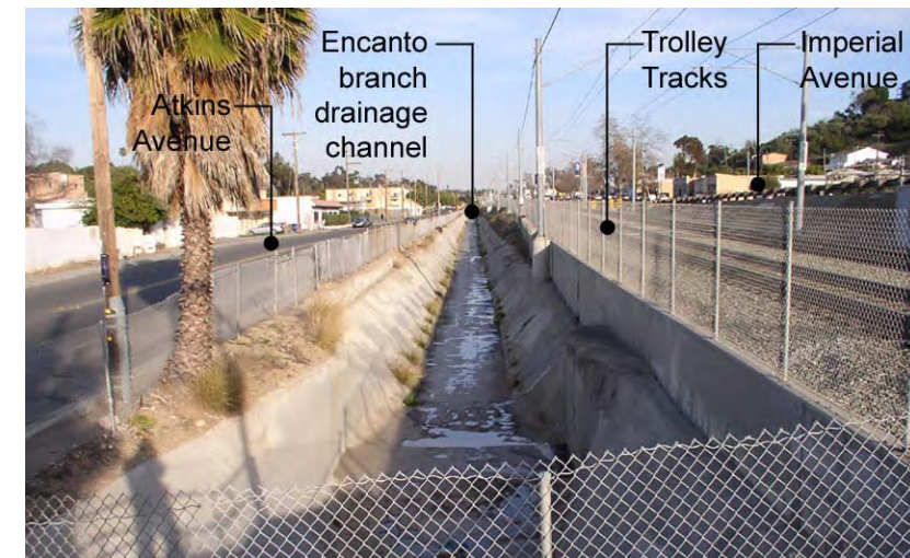
Figure 6.3 - Existing Drainage Channel
