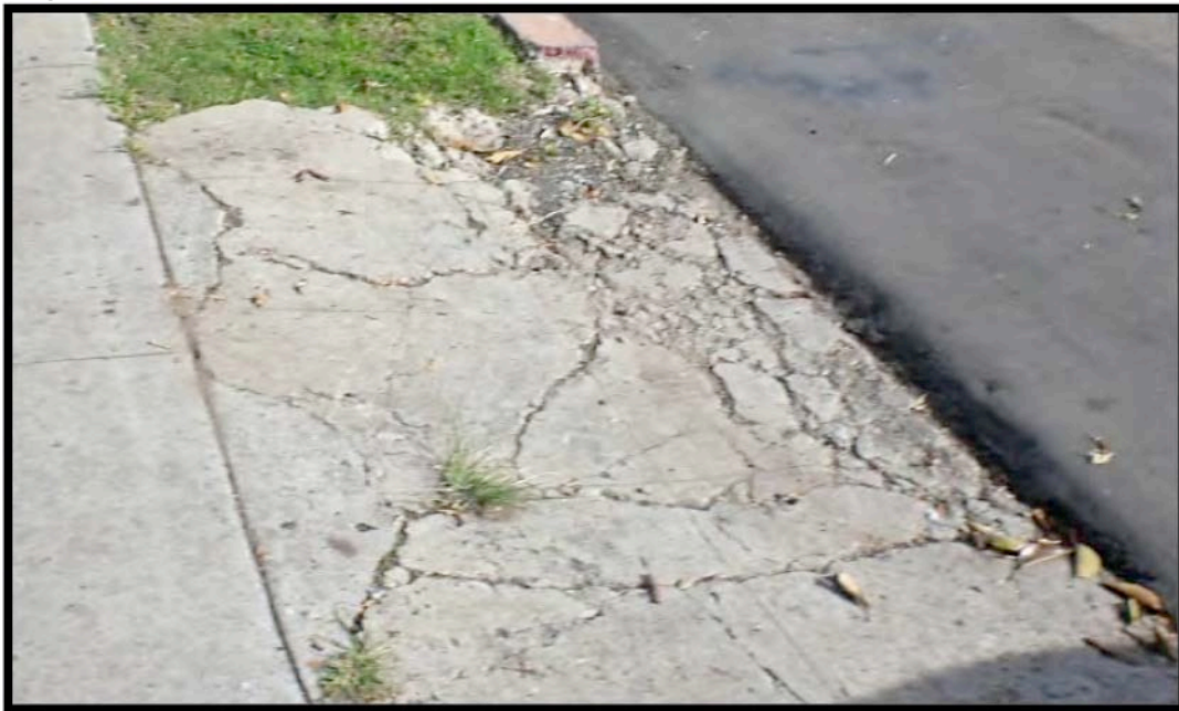
Figure 11.03: Cracked Pavement
