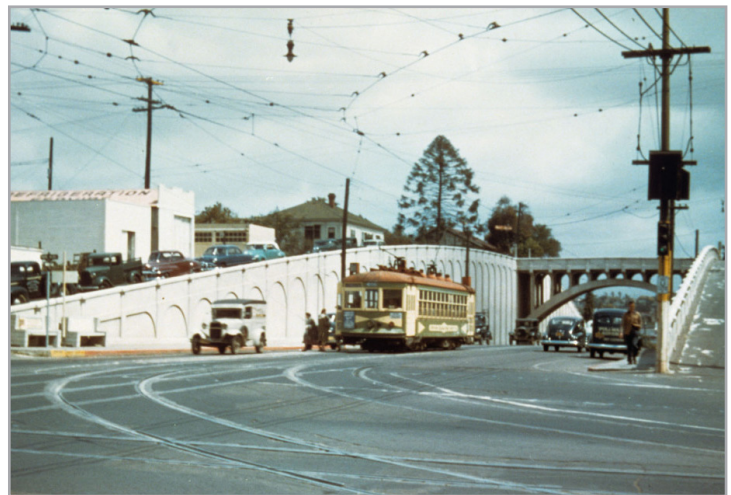
No longer having to traverse the ridge bisecting Hillcrest from North Park, the Georgia Street Bridge was a crucial transportation link when constructed in 1914. This parabolic hinged-arch naturally served as a means for streetcars to connect San Diego with North Park and beyond. The image above at University Ave and Park Blvd (then 12th Ave) portrays this local landmark during the late 1940's.
