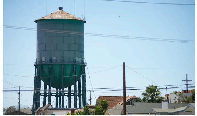
The University Heights Water Storage and Pumping Station Historic District is listed on the National Historic Register of Historic Places.
