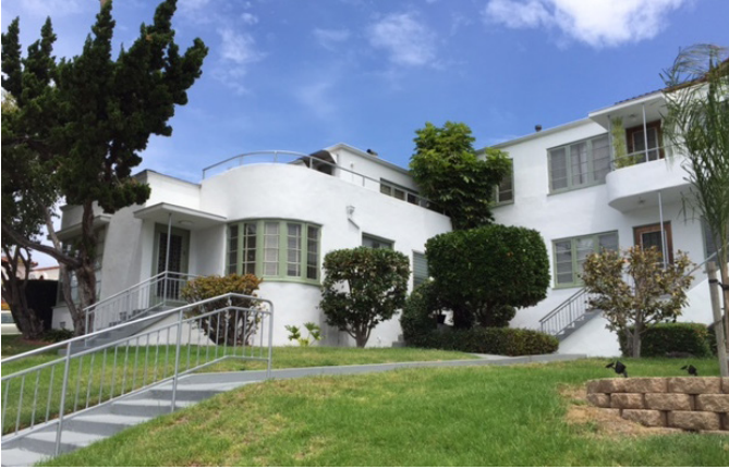
1910 Robinson Avenue built in 1937 characterizing the Streamline Moderne architecture style, is a potentially significant individual resource identified in the 2015 North Park Historic Resource Reconnaissance Survey.
