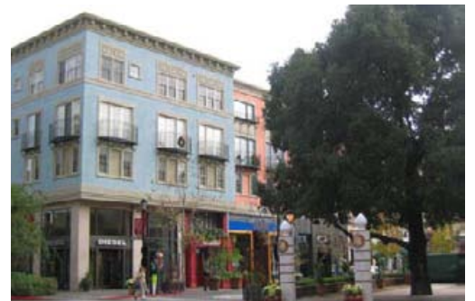
Figure 4.3d - Example of Multi-Family Residential over ground floor retail, using a variety of window types, balconies, and horizontal and vertical plane breaks to help create a village character.
