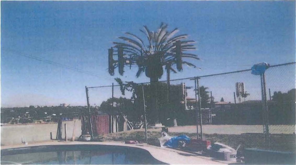
View of Monopalm and T-Mobile antennas looking from West to East
