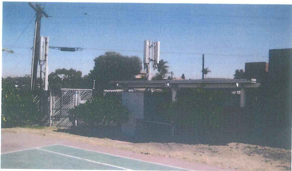
Existing T-Mobile Antennas and Equipment (Garden Shed to the Right)
