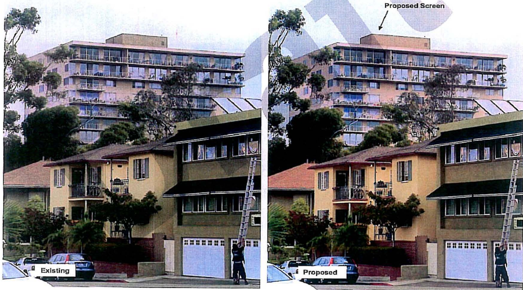
SAN-010 Coral Tree Plaza - Photosimulation of Proposed FLO TV Site Photo Looking North-East from 6 th & Ivy
