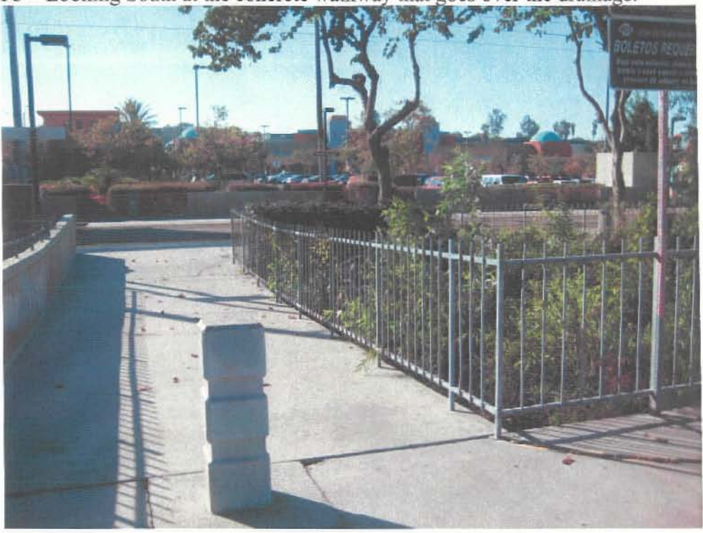
P3 – Looking South at the concrete walkway that goes over the drainage.
