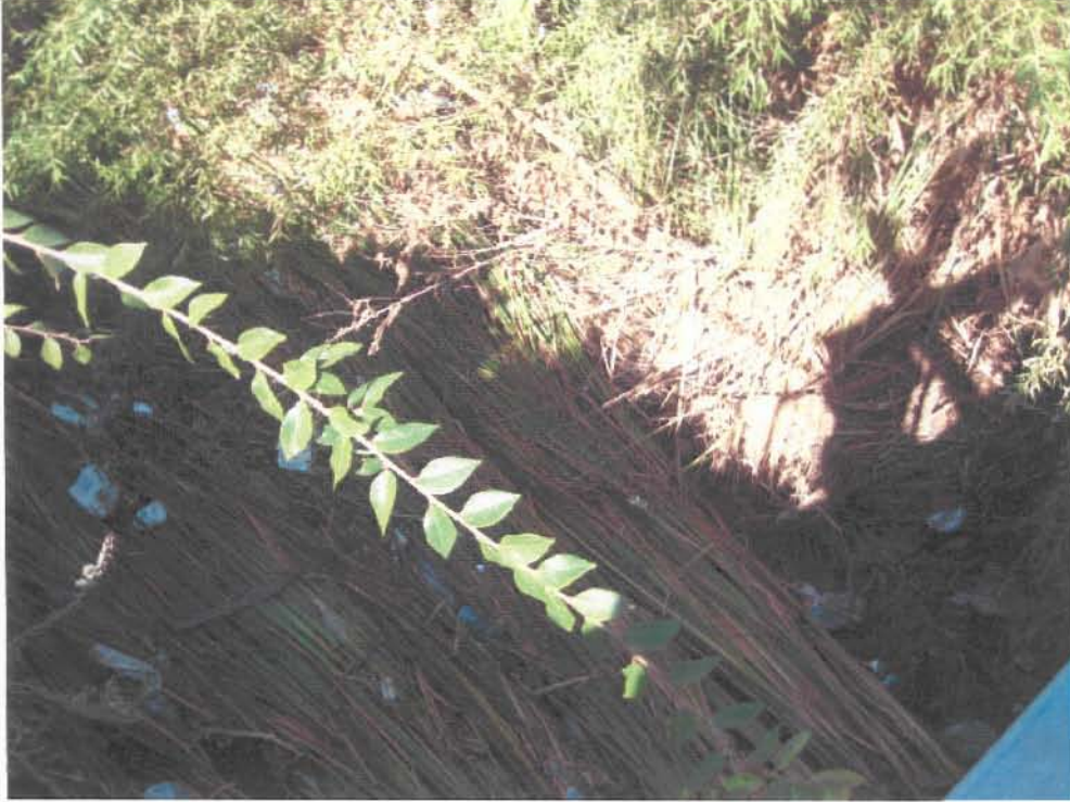
P1 – Looking down into drainage area towards the location of MH 88
