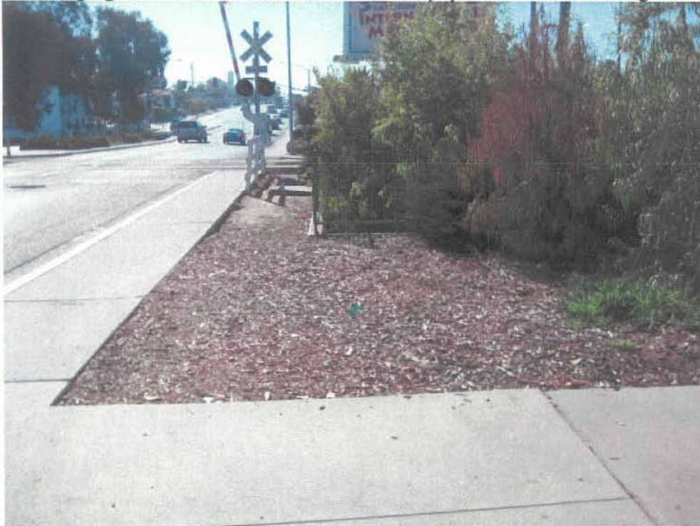
P2 – Staging area for the crane that will lower equipment into the drainage area.
