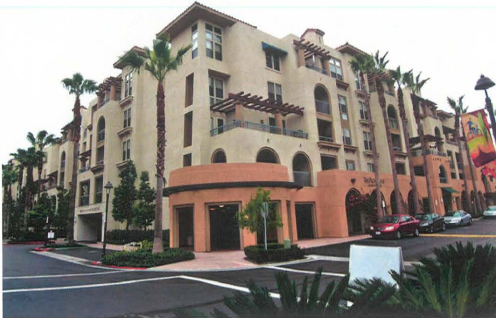
1) Typical of exterior finishes at Building 4.
