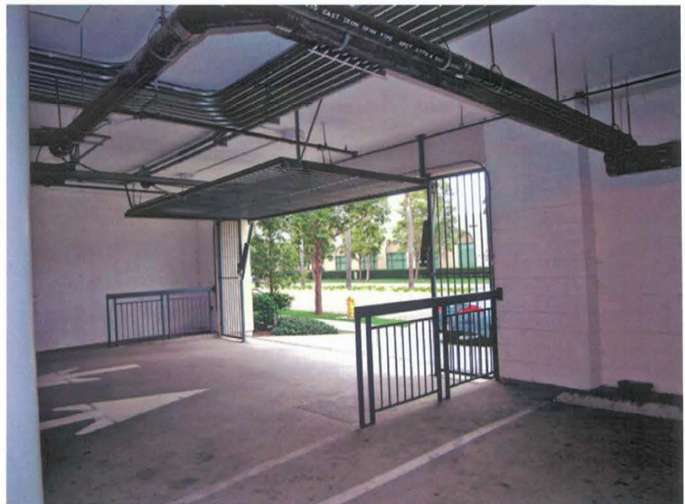
10) Typical of parking garage exits
