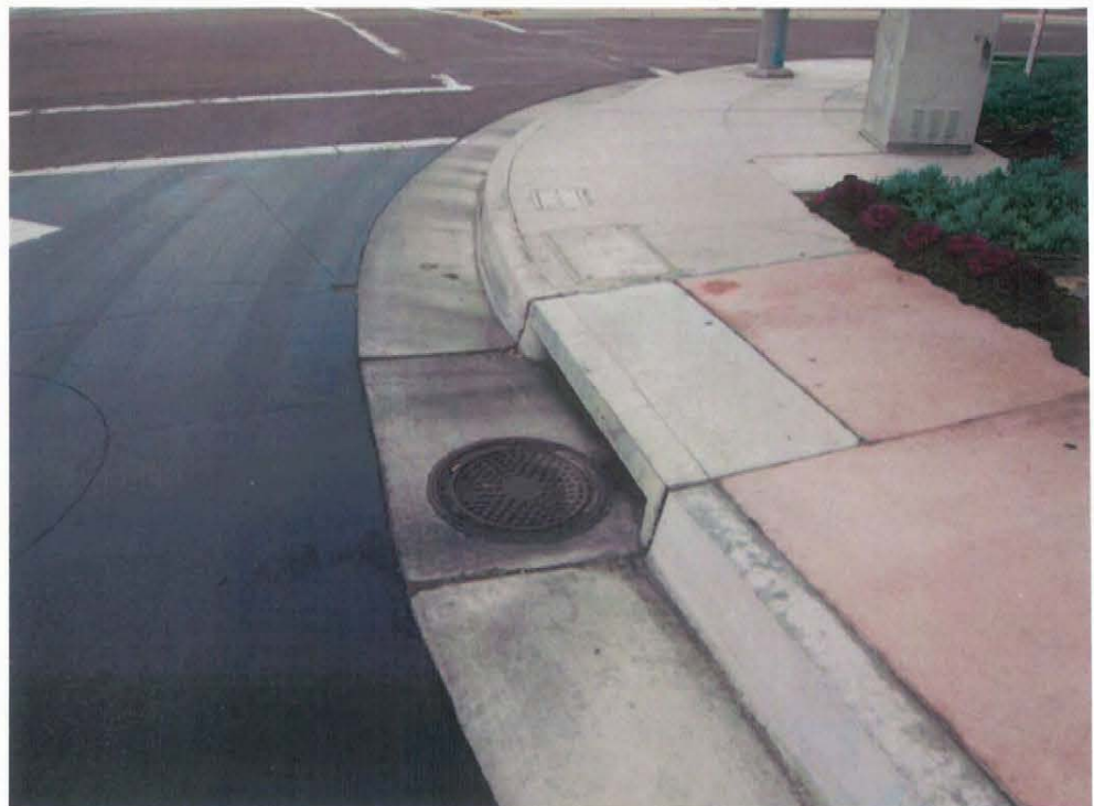
6) View of storm drain inlet.
