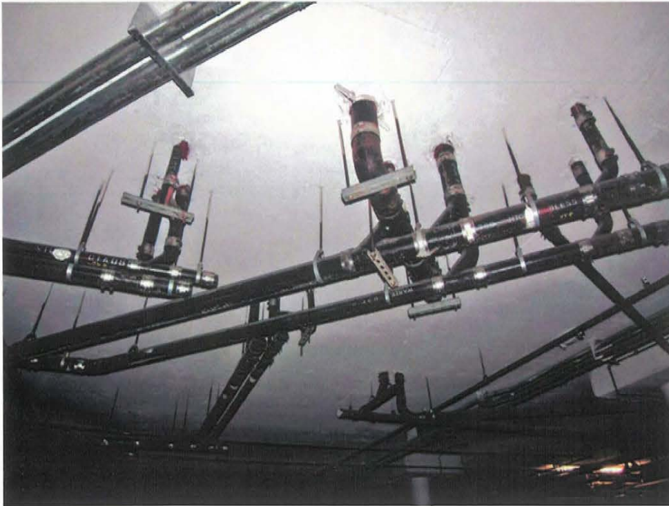
11) Typical of cast iron sewer waste piping visible in parking garage.
