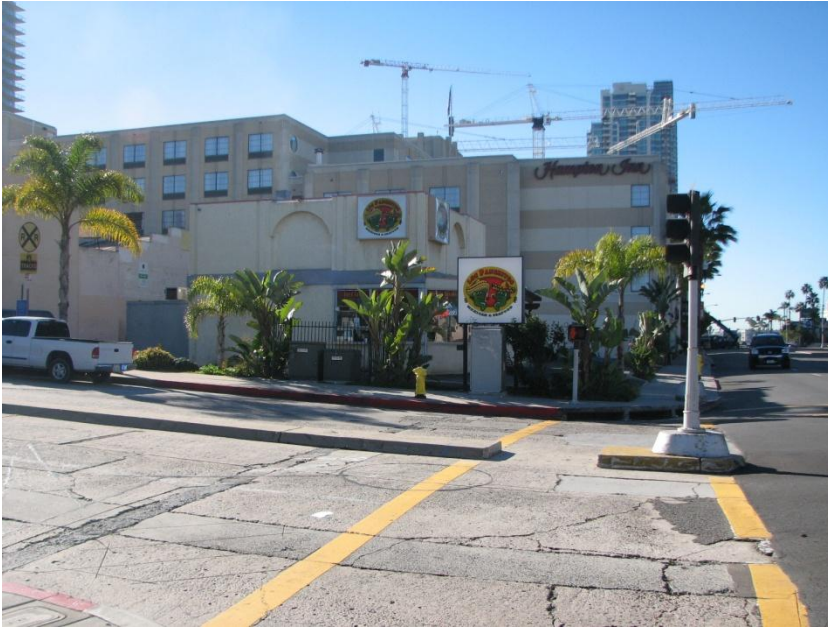
View of site's north face from Cedar Street
