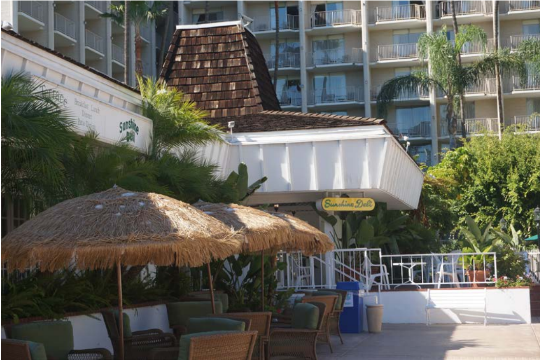
Plate 31. Terrace Café pavilion roof form with wood shingles
