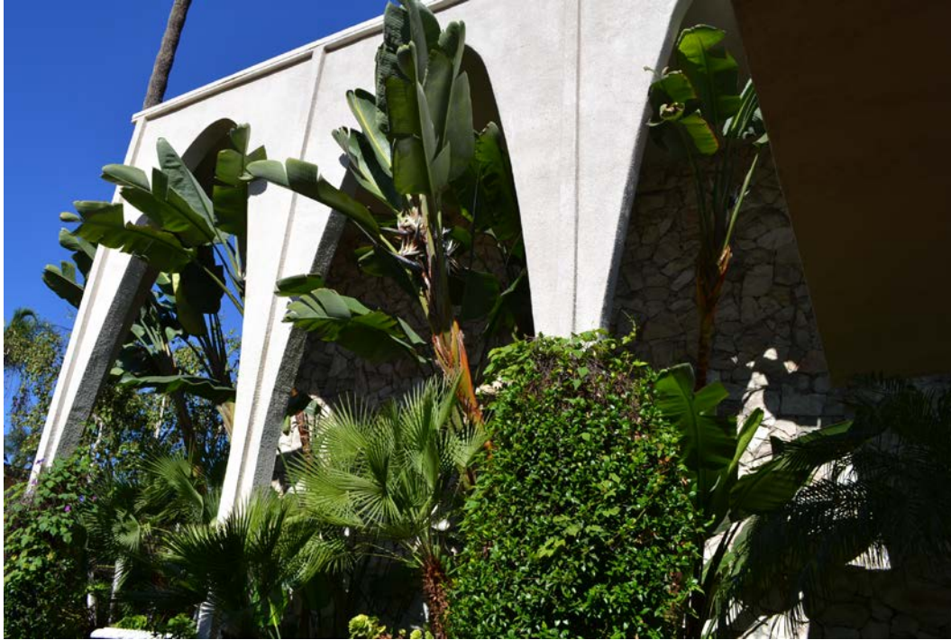
Plate 34. Parabolic arch loggia and stone exterior wall siding, Regency Conference Center
