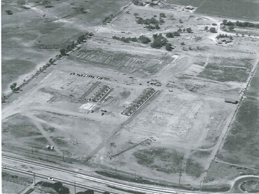
Construction. Aerial, looking north (1953 San Diego History Center)
