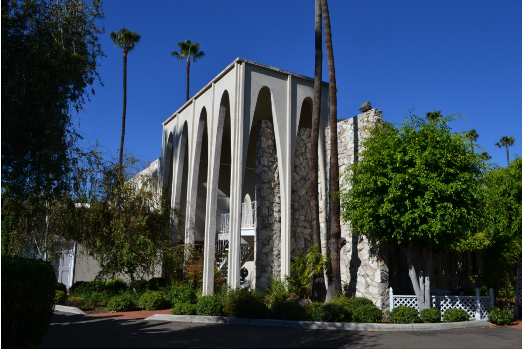
Plate 24. Bldg. 3600, south façade facing Hotel Circle North
