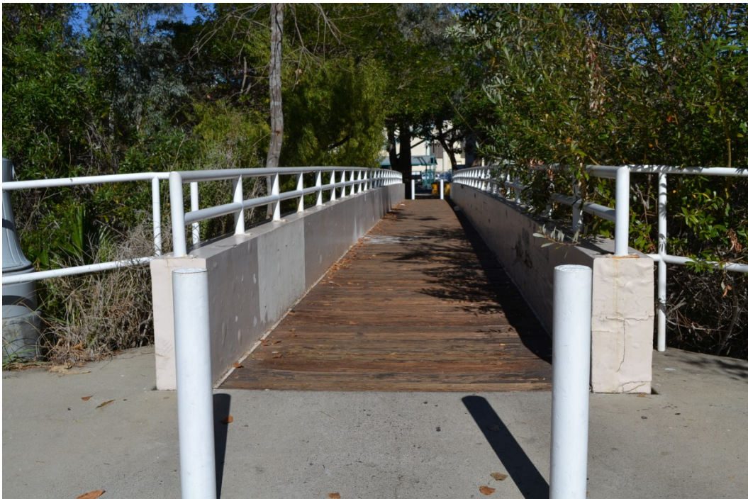
Plate 29. Pedestrian bridge crossing the San Diego River to Fashion Valley
