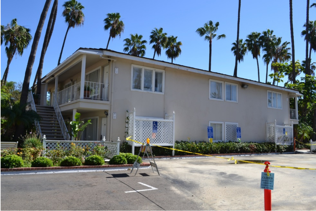
Plate 20. West elevation of center building in Bldg. 3500 complex
