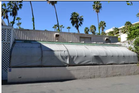
Maintenance Building, Gardening Storage
