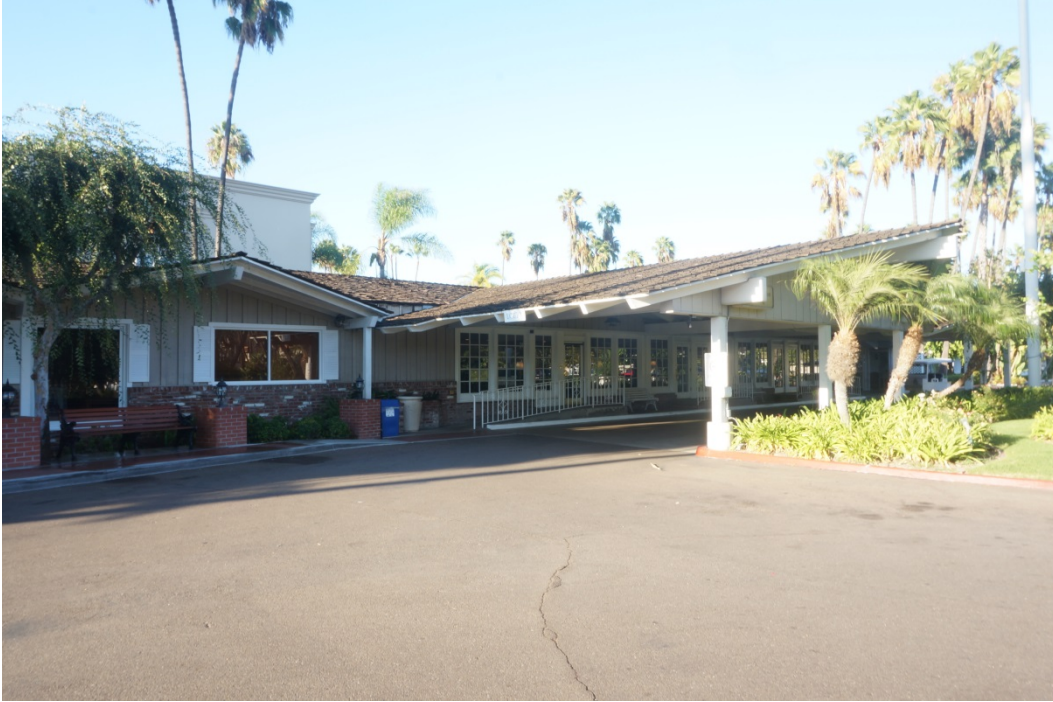
Plate 18. Lobby and porte-cochere with exposed framing
