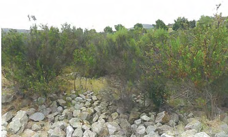
Figure 8: Basin 900/1000 Reach 3 – Standing in Channel, Looking Downstream
