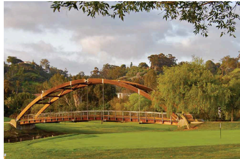
Existing pedestrian bridge to be retained within Riverwalk
