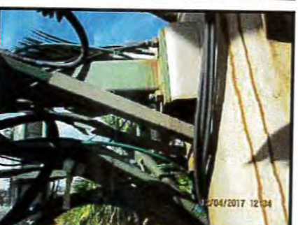
#7 Antenna Mount Connection
