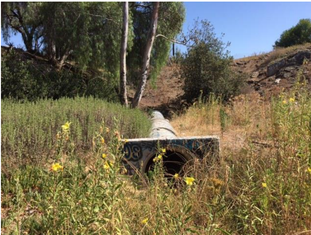
Photo 2. Culvert in unnamed drainage facing south.
