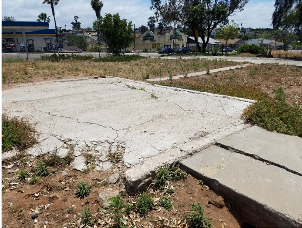
Photograph 3. Detail of foundation along Euclid Avenue, facing southeast.
