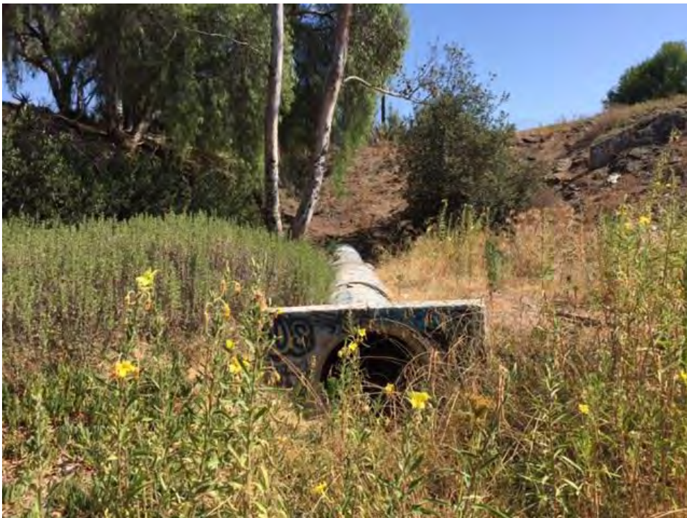
Photo 2. Culvert in unnamed drainage facing south.
