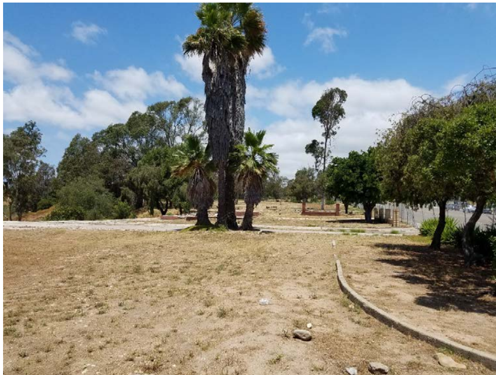
Photograph 2. View of foundations and driveways along Euclid Avenue, facing north.
