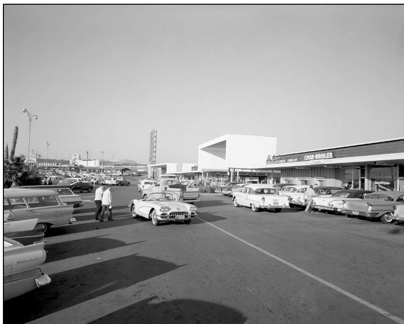
Figure 35. Clairemont Quad Shopping Center (1959). Source: San Diego History Center
