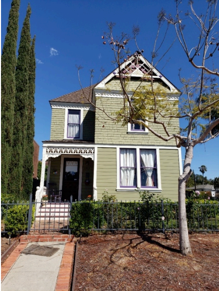
Figure 8. The Stough-Beckett Cottage, designated as HRB No. 146 and located at 2203 Denver Street. The home was previously addressed as 3003 Denver Street.
