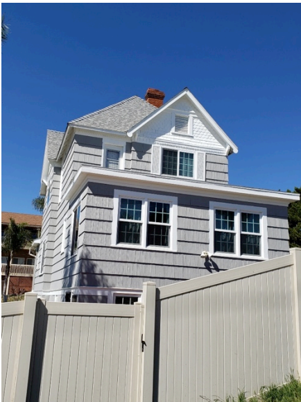
Figure 10. The Ambort Residence, located at 4440 Ingulf Street. The home was previously addressed as 4240 Ingulf Street.
