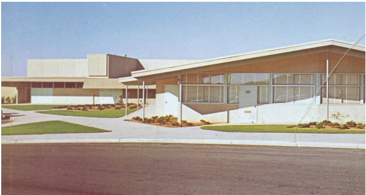
Figure 31. Clairemont High School (1960). Source: Clairemont High School Yearbook
