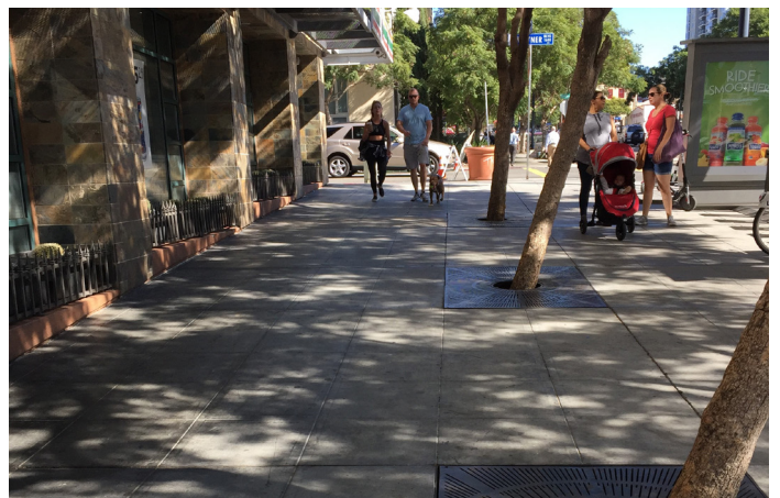
Enhanced sidewalk and landscaping provide an improved pedestrian environment
