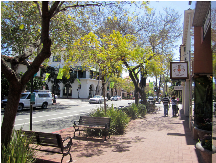
Sidewalks with a furnishing area that incorporates street furniture, street trees, and landscaping help create a comfortable and attractive pedestrian environment.
