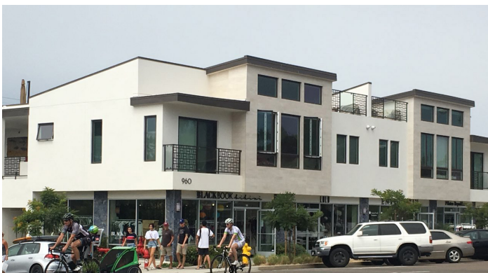
Primary building entrances fronting the street encourage an active public realm.
