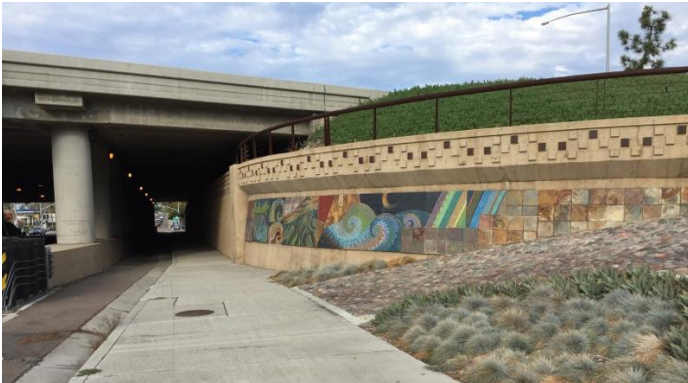
Sample of walkway with enhancements at freeway underpass.
