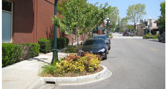
Bulbouts with flow-through planter helps reduce traffic speeds while enhancing the street with landscaping and street trees and stormwater management
