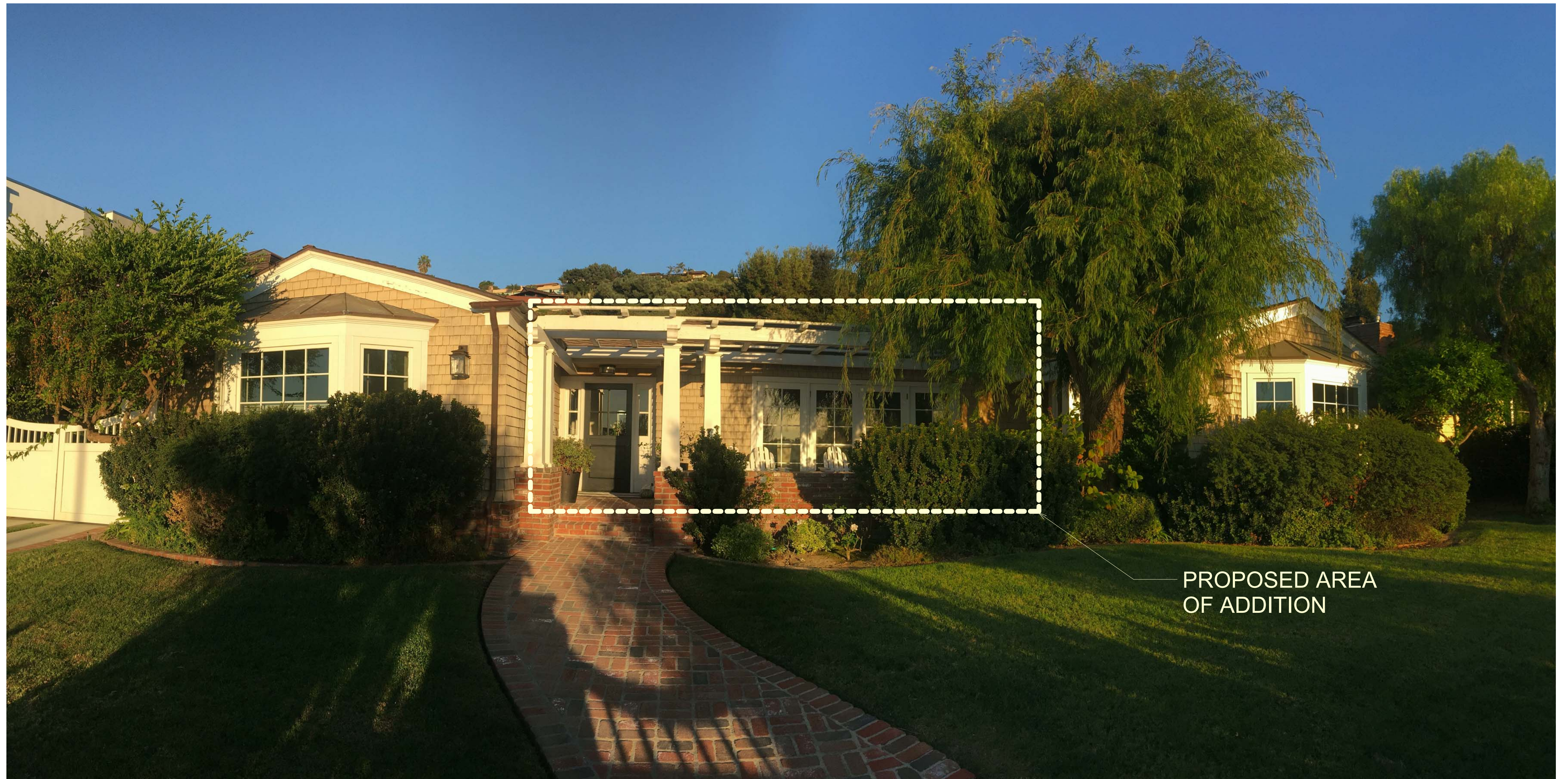
8315 CALLE DEL CIELO WEST ELEVATION FROM YARD
