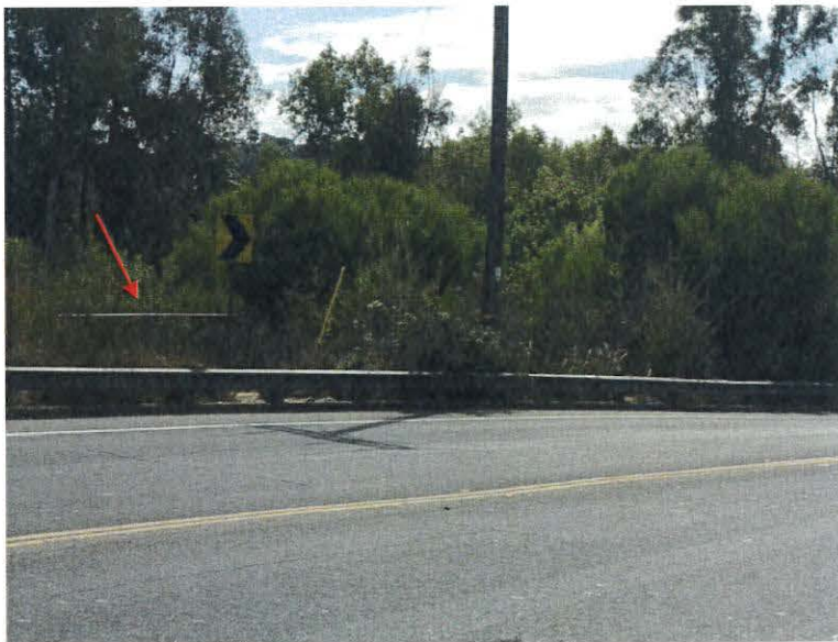
Photo 4. This photo shows the existing chain-link fence that separates the ROW from the riparian habitat within the San Diego River.
