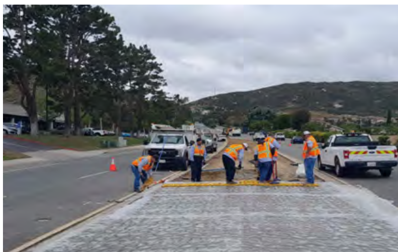
City crews constructing a center median.
