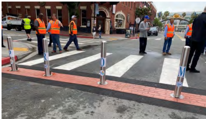
Bollards installation on Fifth Avenue Source: City of San Diego, 2023
