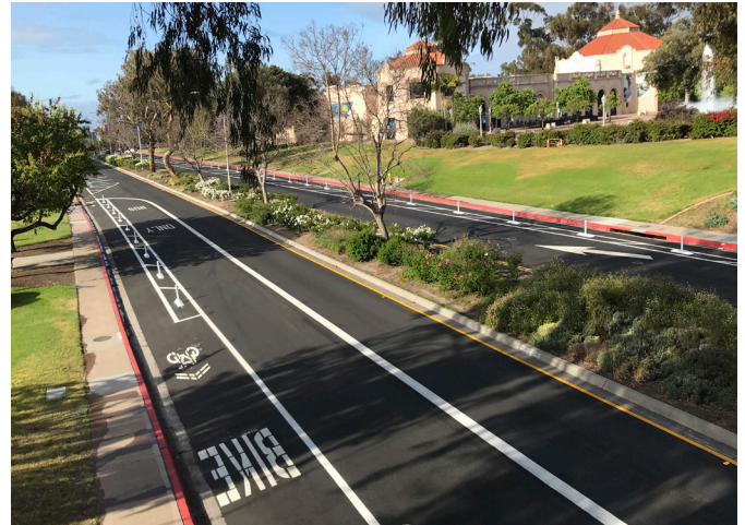
Road resurfacing with multimodal facilities on Park Blvd Source: City of San Diego
