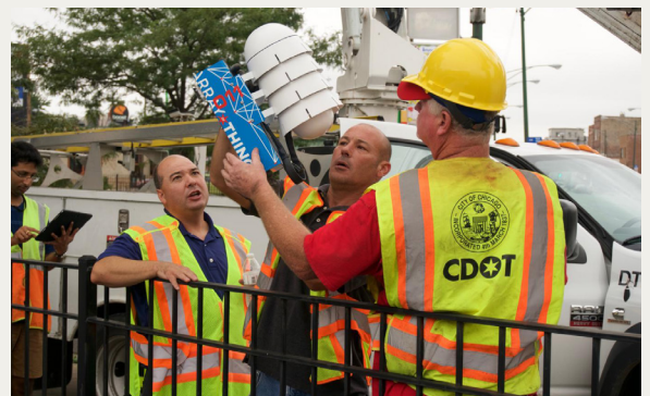
Installing AoT sensors, Chicago Source: University of Chicago, 2016
