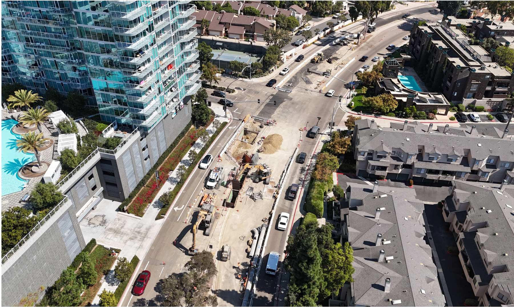
Pipeline construction along Nobel Drive
