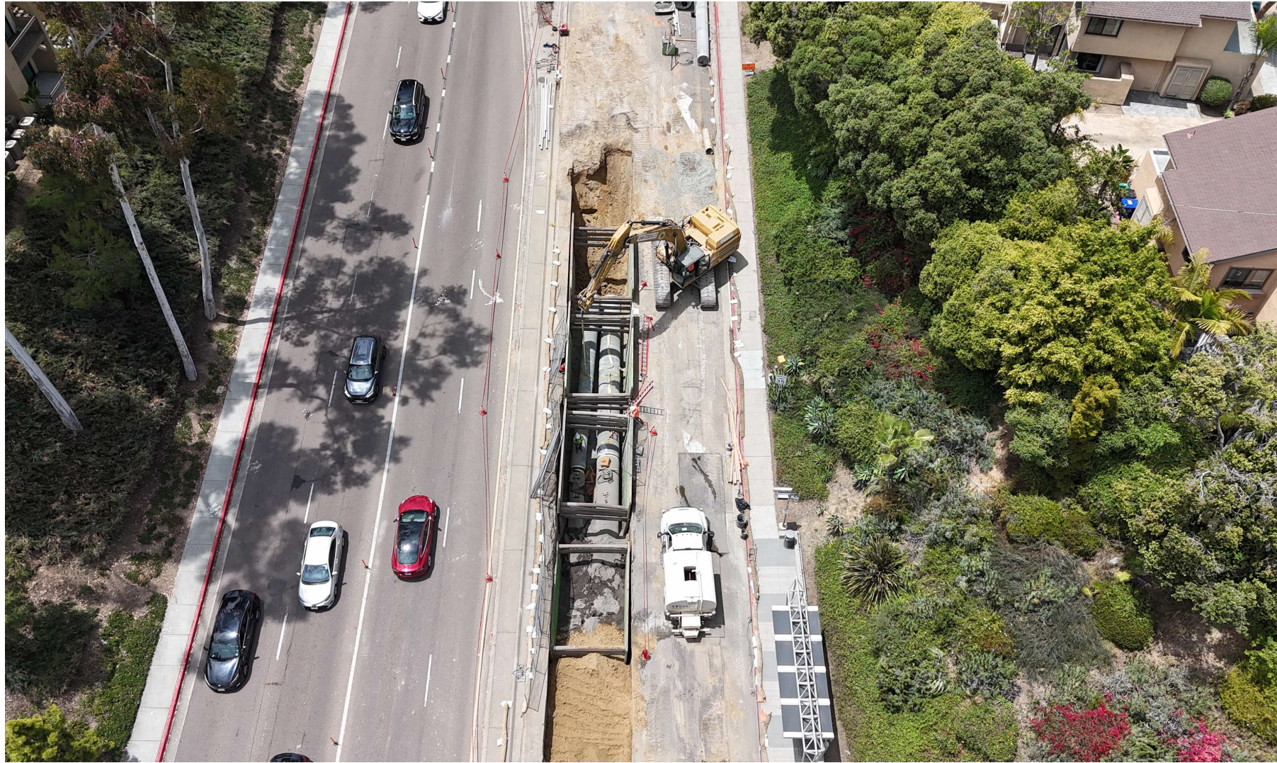
Pipeline construction along Nobel Drive
