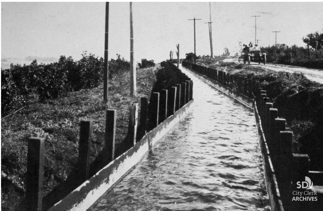
Figure 4: An example of the open flume at an unknown location in 1905 as built by the San Diego Flume Company. Image Source: San Diego City Clerk's Office.
