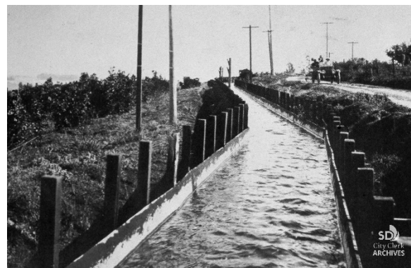
Flume to transport water to San Diego from Cuyamaca Mountains, 1905, City of San Diego City Clerk's Archive
