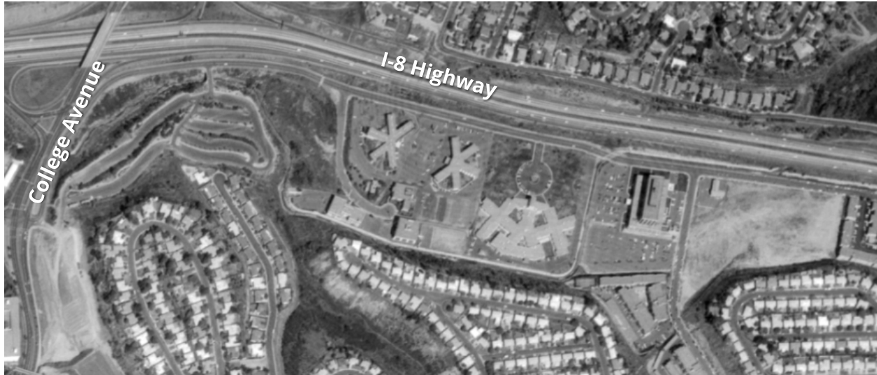
Figure 59. Aerial photograph from 1974 showing the area that had developed as the Alvarado Medical Center and Hospital in the 1960s. Source: Flight AML-SD, Frame 7017, February 1974. Courtesy of UCSB Library Geospatial Collection.
