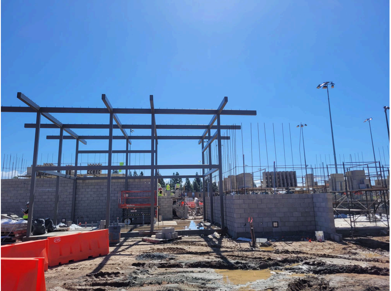
Aquatic and Equipment Buildings CMU block installation.
