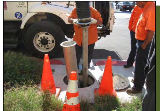
Insertion of vacuum hose into separation chamber.
