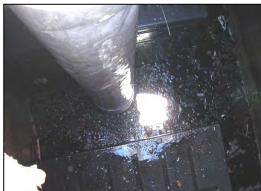
Removal of trash, sediment and debris.
