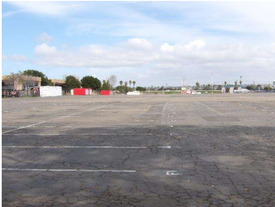
Photograph 3: Overview of CA-SDI-10530H, southwest parking area, facing north.
