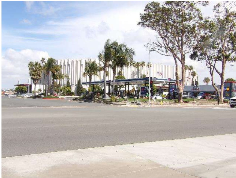
Photograph 11: P-37-035181 (San Diego Sports Arena) behind ARCO station, facing north.
