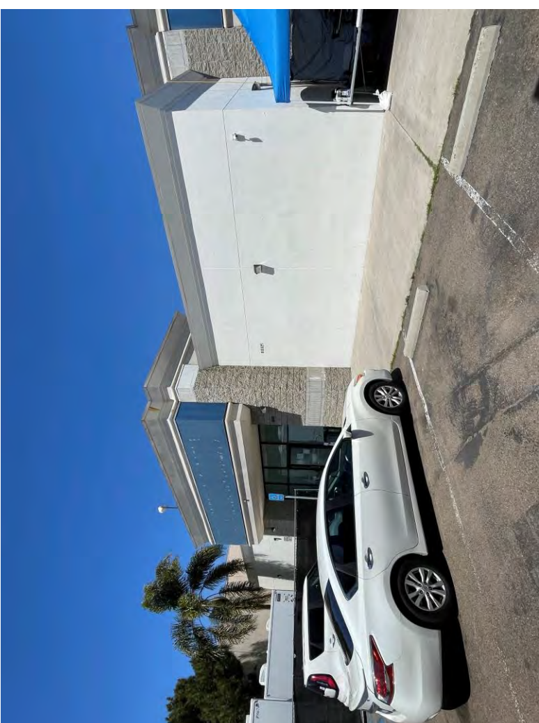
South Elevation; View Facing West
