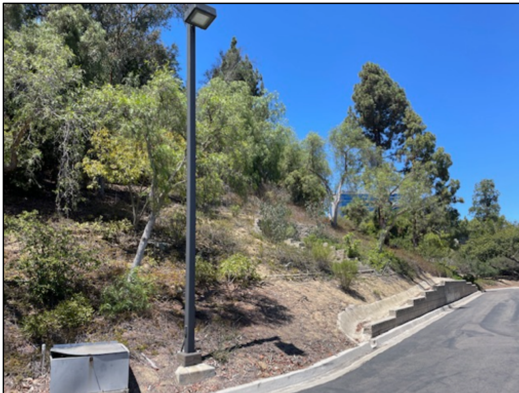
Photograph 4. Urban/Developed parking lot and retaining wall with Ornamental Plantings on manufactured slope along the northern perimeter of parking lot (taken 8/3/21; facing east).
