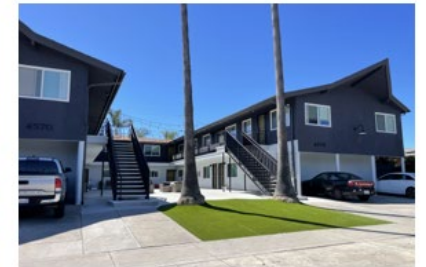
Figure 107: Apartment building (4570 Wilson Avenue, built c.1953-64) with a projecting peaked roof and tuck-under parking.
