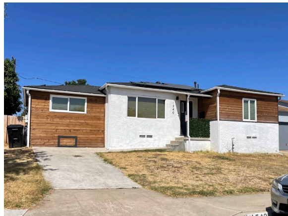
Figure 9. An example of an altered Postwar Minimal tract home in Arnolds Park.
