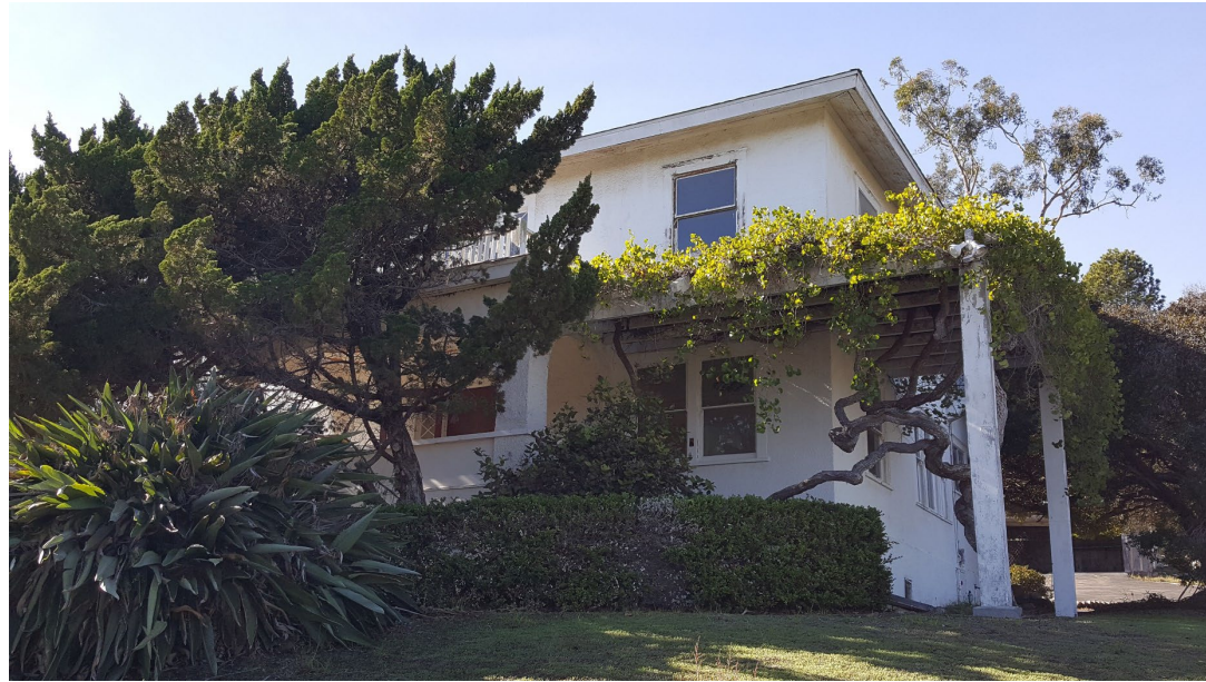
East Elevation; View Facing West
