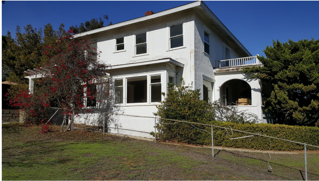
South & East Elevations; View Facing Northwest
