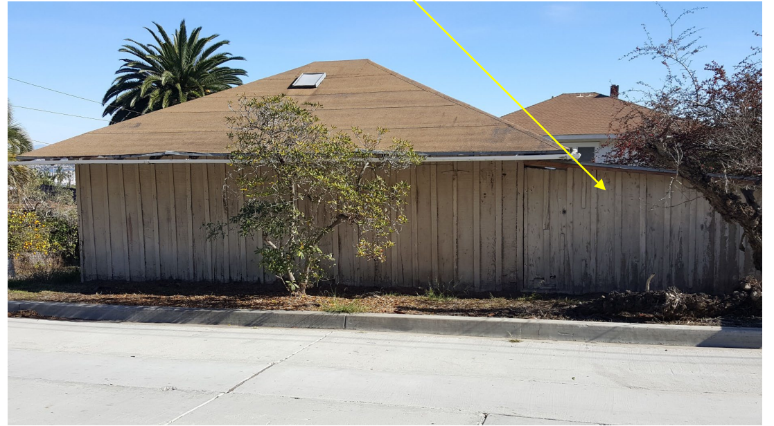
Note Shed Addition (Right)
