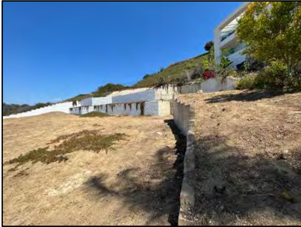
Plate 3: Overview of the terraced retaining walls, facing northeast.
