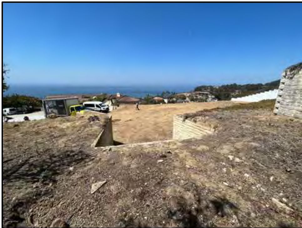
Plate 4: Overview of the project from the terraced retaining walls, facing north.
