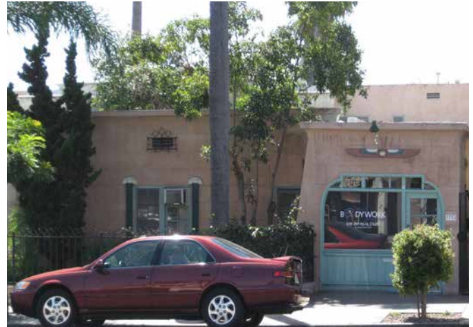
Egyptian Courts Apartments, built in 1925, are located along the Egyptian thematic corridor along Park Boulevard.
