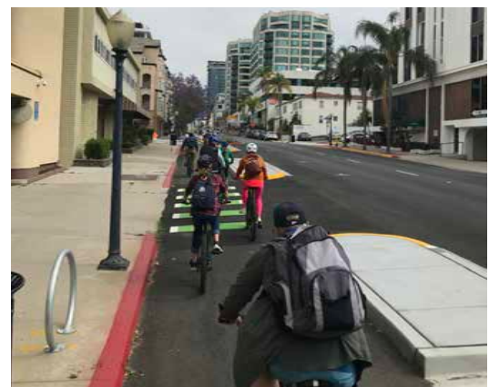
A cycle track along Fifth Avenue connects Downtown with Bankers Hill/Park West and Hillcrest.
