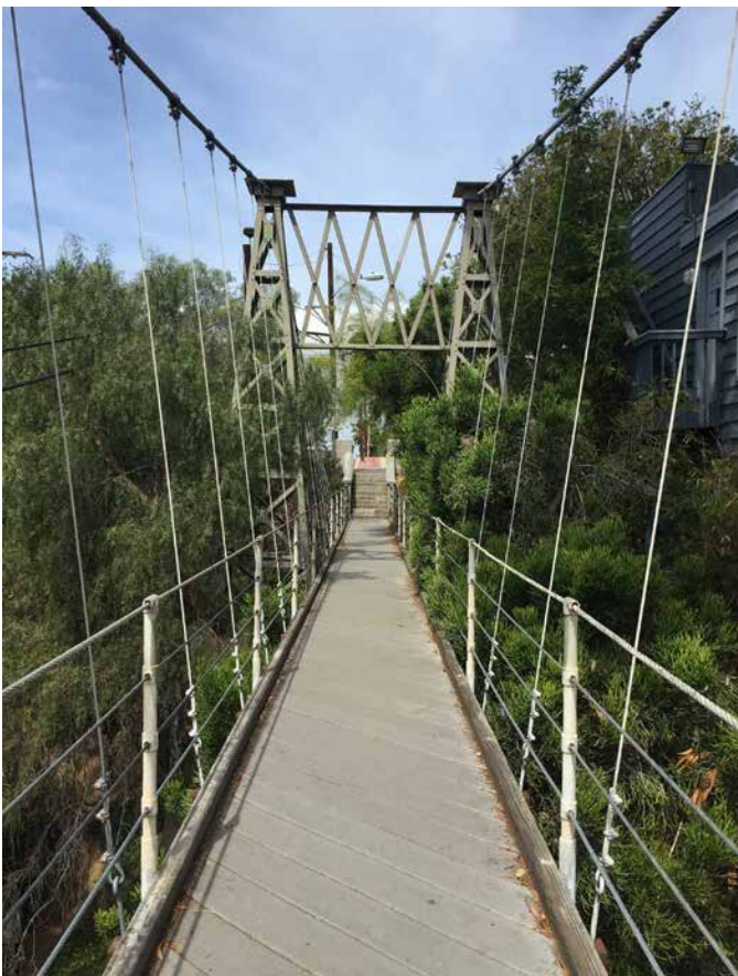
The Spruce Street Bridge, engineered by Edwin Capps, still provides access over ArroyoMaple Canyon since its completion in 1912.
