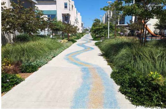
Example of a pattern treatment type: glass seeded concrete
