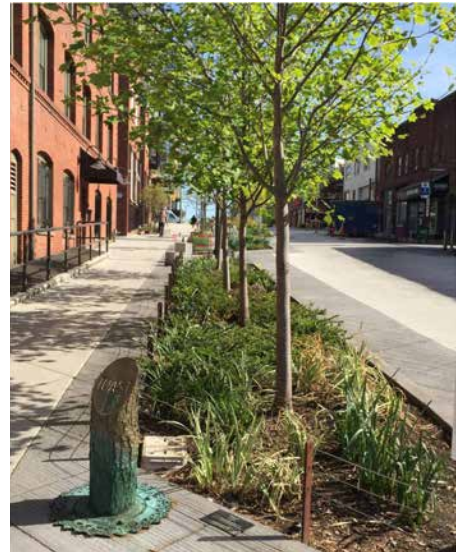
Bioswales along streets can serve the dual function of creating aesthetically pleasing urban areas and filtering storm water.
