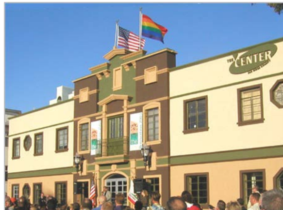
The Center, 3909 Centre Street, 2016 Source: Hillquest, http://www.hillquest.com/recreation/urban-walk-2-university-avenue-east/ .
