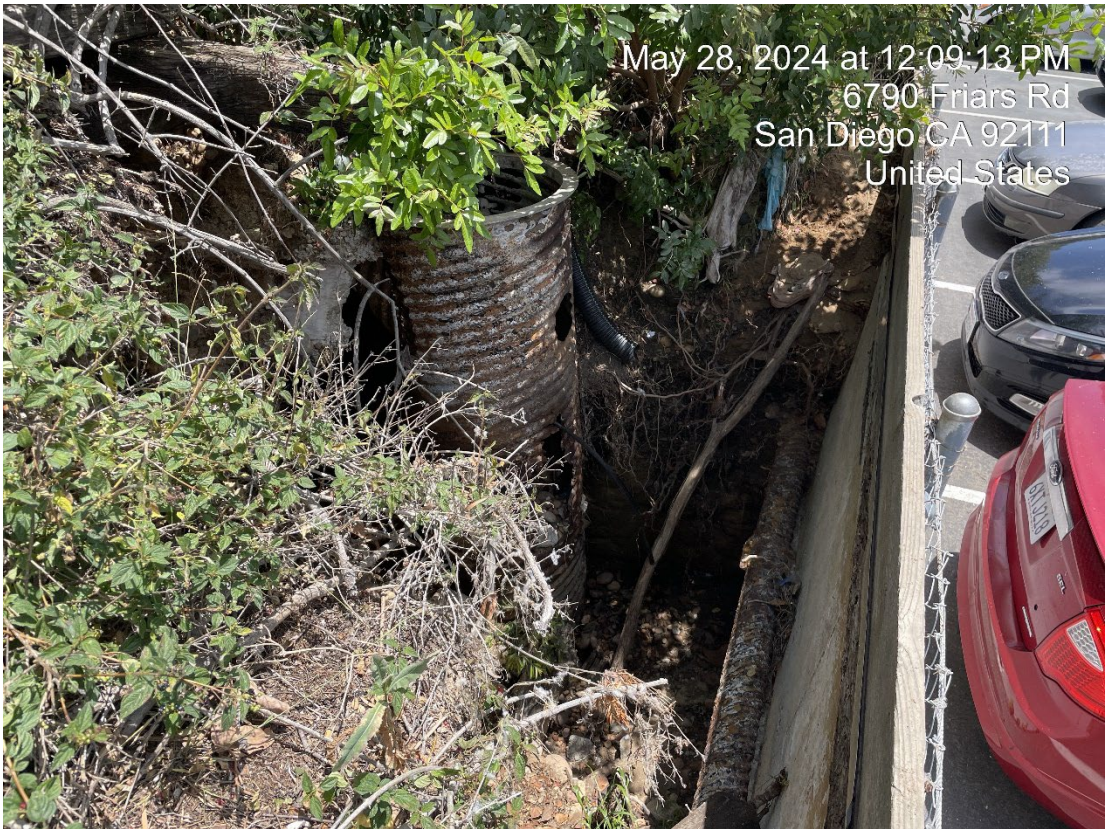
CMP riser draining from corroded connection
