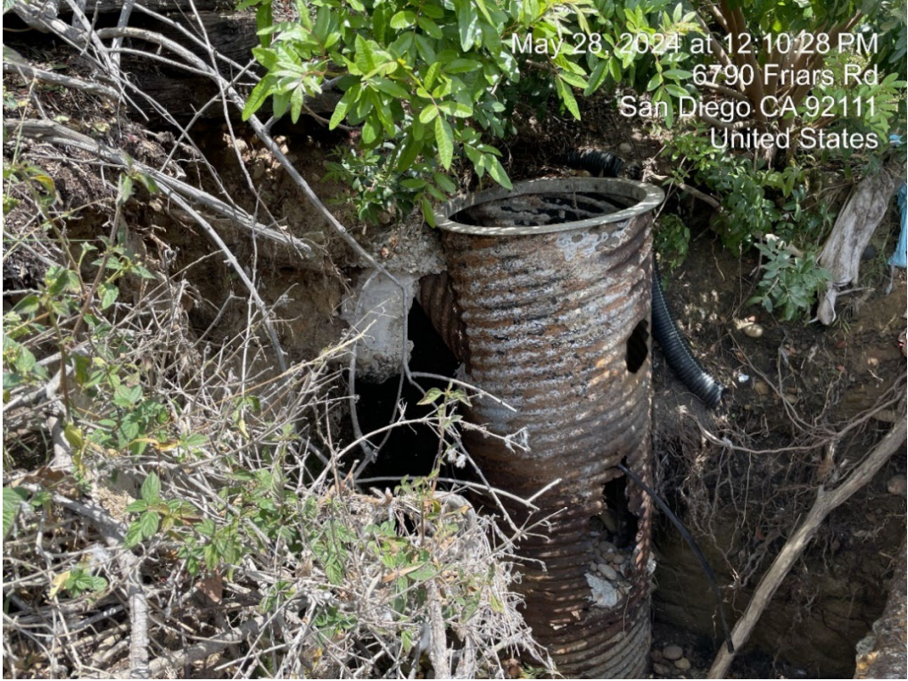
CMP riser draining from corroded connection
