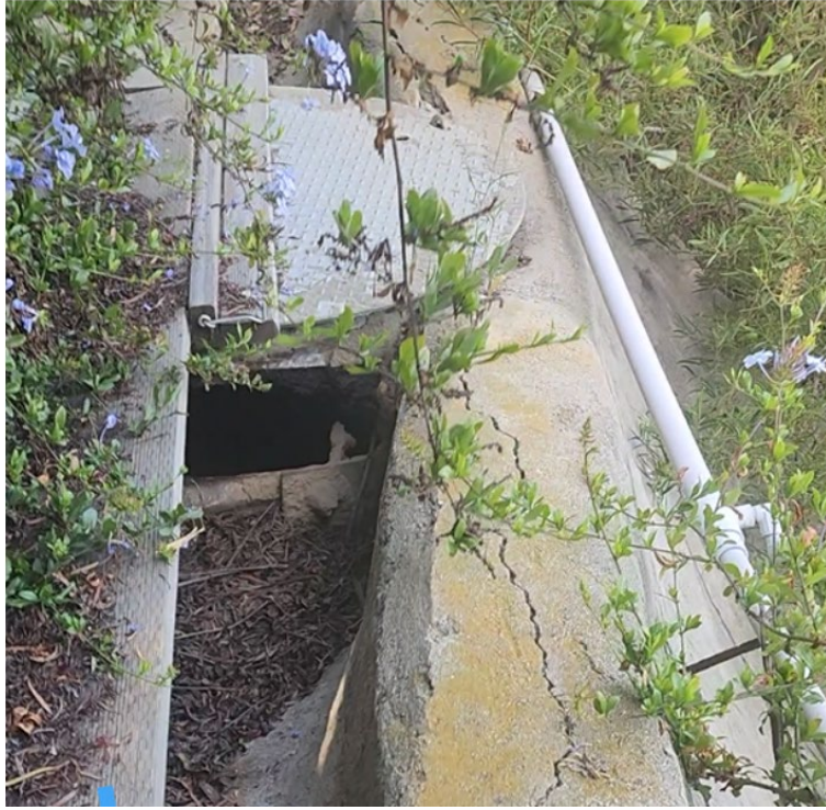
Upstream modified CMP riser
