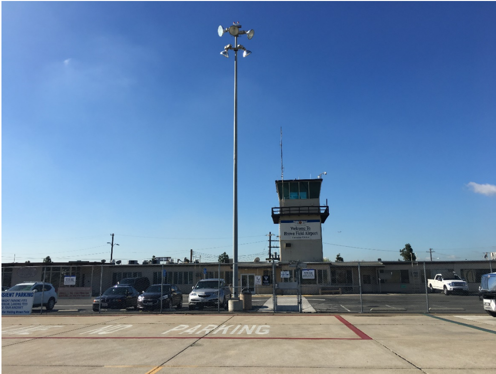
View of Former Air Traffic Control Tower and Terminal Building.
