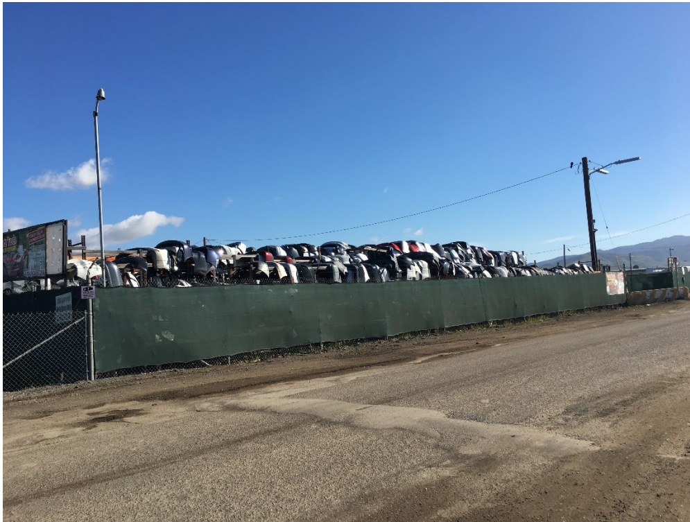
View of auto auction/wrecking yard on north portion of the Site.
