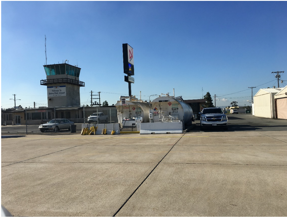
View of ASTs and dispenser at the Terminal Building.
