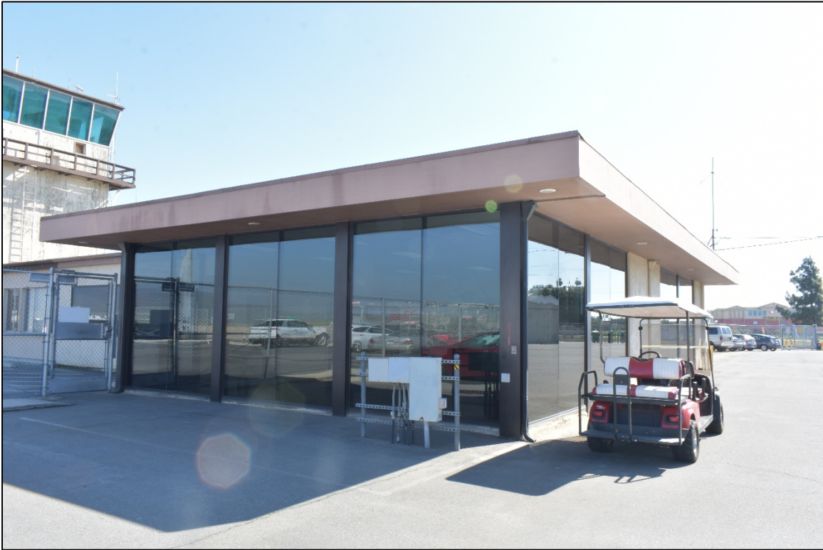
Figure 16: Western end of Building 2002, looking southeast. IS Architecture, 2019.
