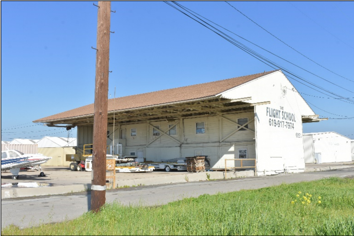
Figure 21: Building 10, looking east. IS Architecture, 2019.
