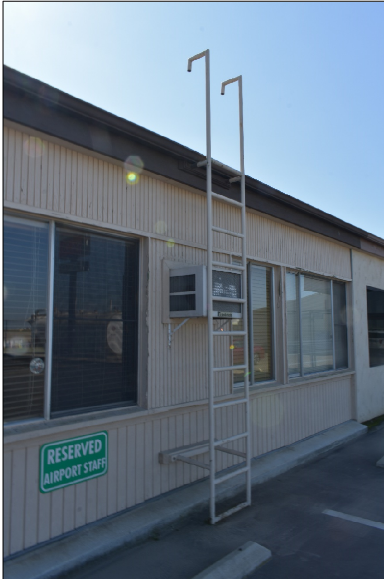
Figure 13: Continuing along the north elevation, west of Fig. 11. IS Architecture, 2019.
