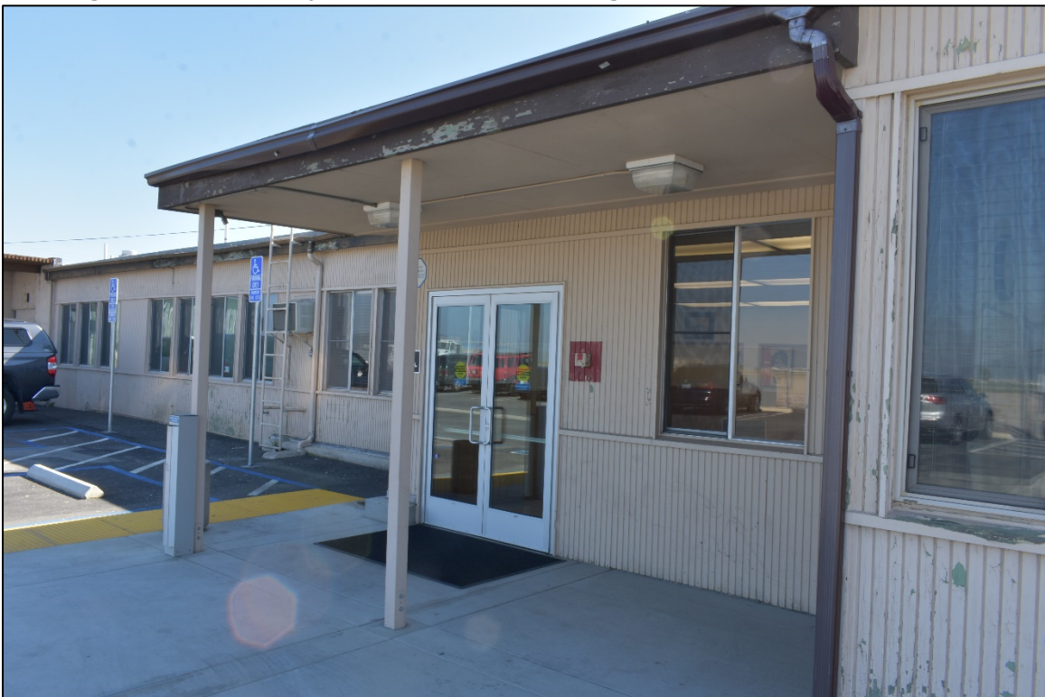
Figure 10: Continuing along the north elevation, west of Fig. 9. Northern entrance (through double doors) of the building. IS Architecture, 2019.
