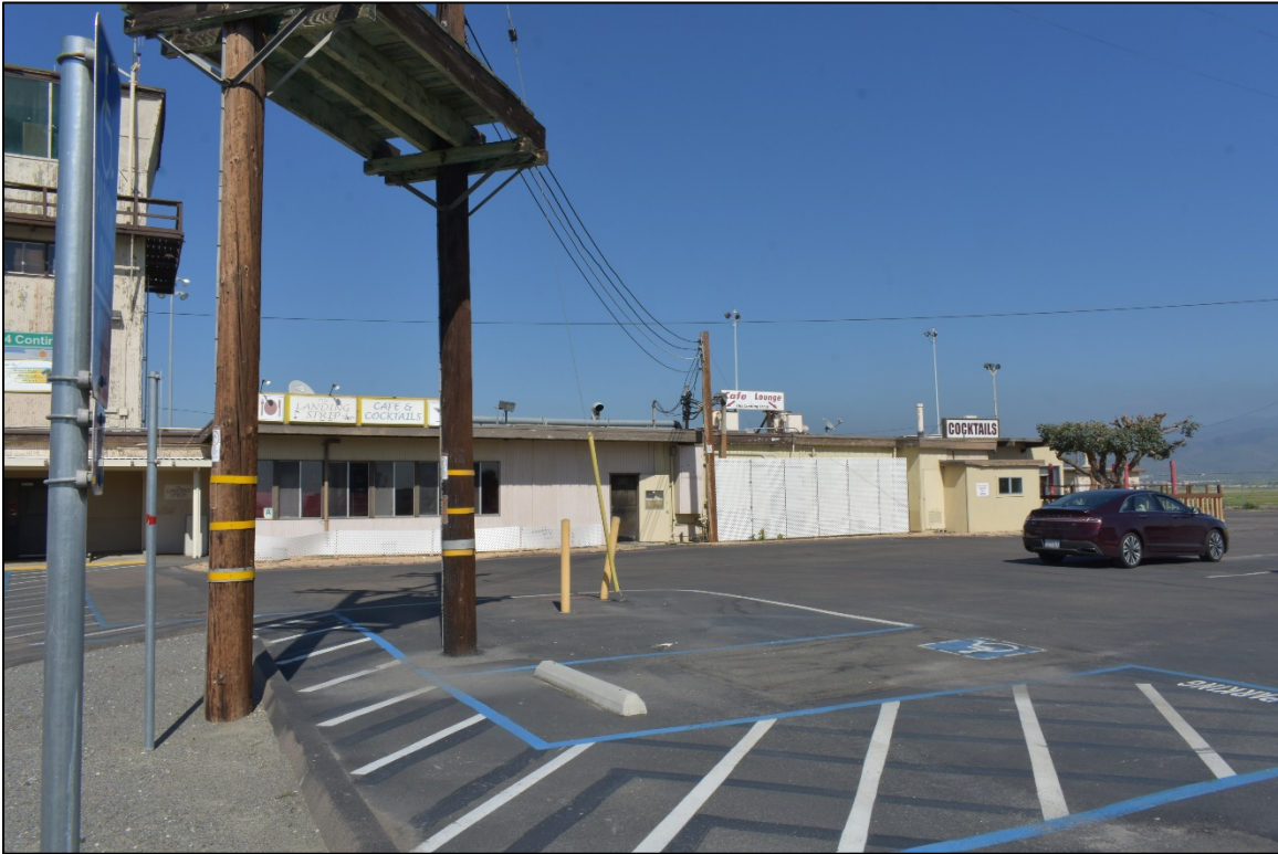
Figure 7: Eastern portion of the south elevation of Building 2002. IS Architecture, 2019.
