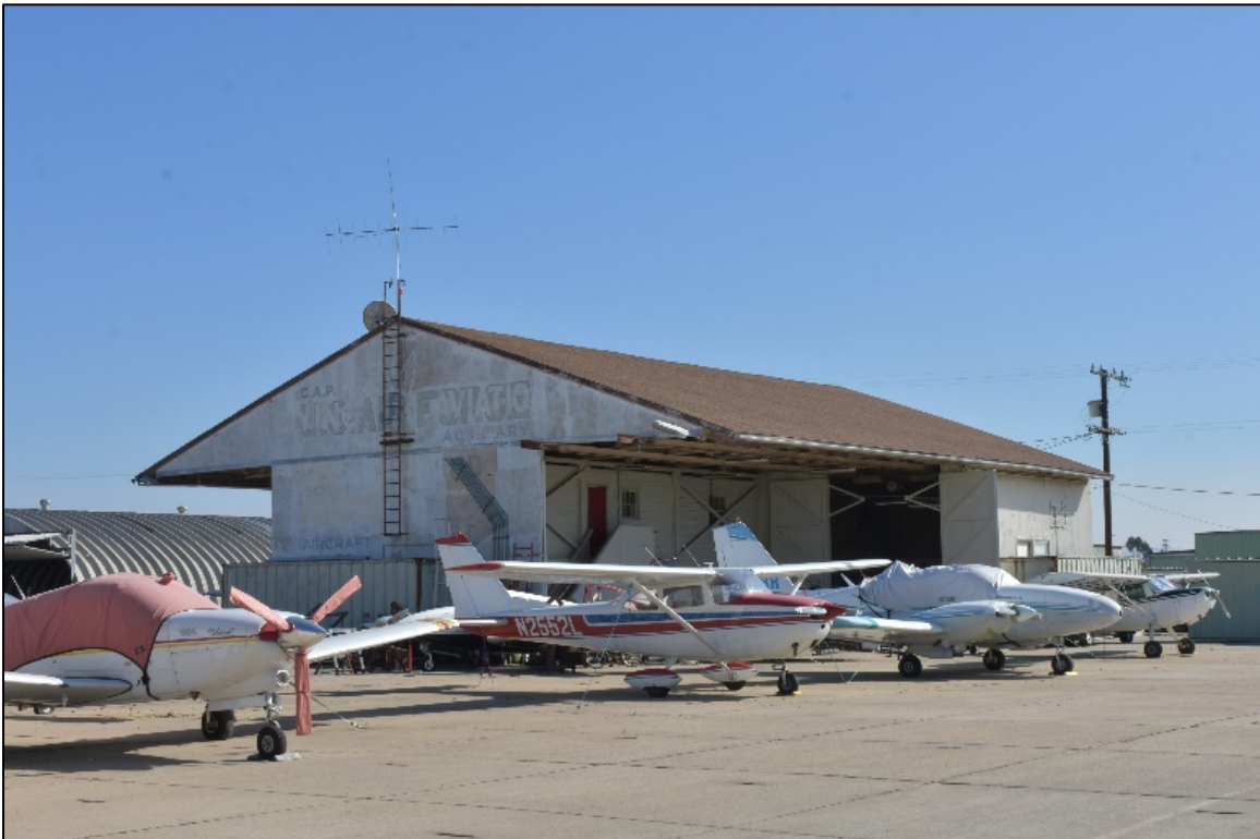
Figure 22: Building 2005, looking south. IS Architecture, 2019.
