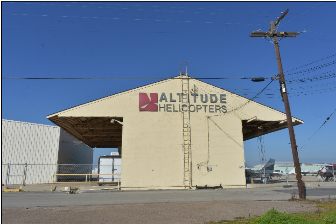
Figure 19: Building 2003, looking north. IS Architecture, 2019.
