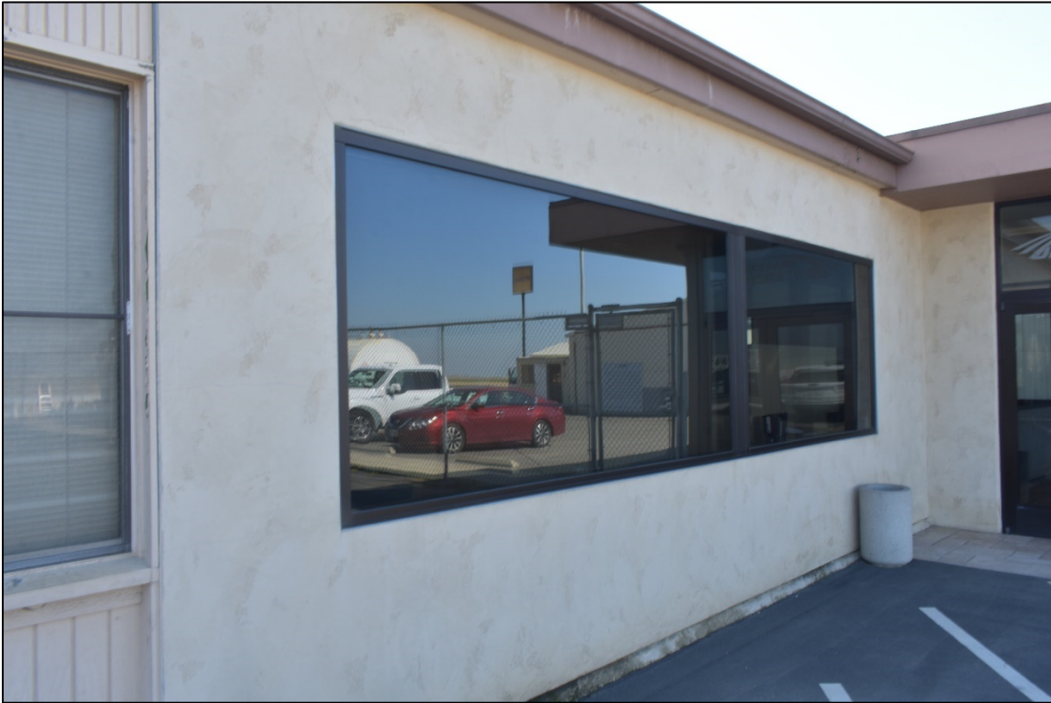
Figure 14: Continuing along the north elevation, west of Fig. 13. IS Architecture, 2019.
