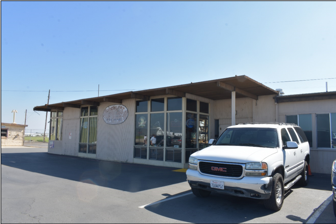
Figure 9: Eastern end of the north elevation, looking southeast. IS Architecture, 2019.
