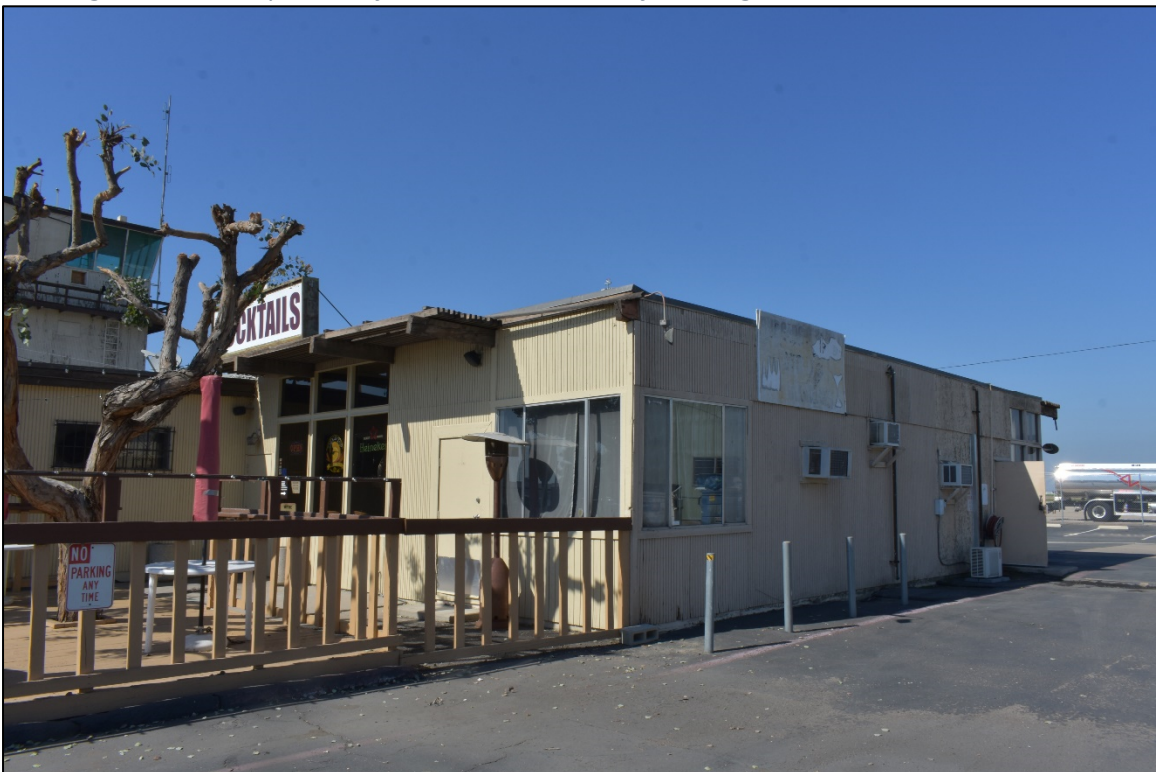
Figure 8: Eastern end of Building 2002, looking northwest. IS Architecture, 2019.
