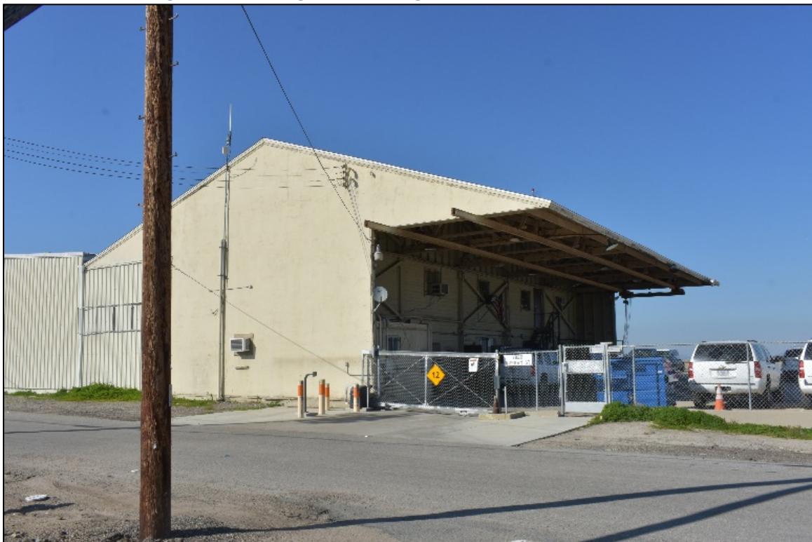
Figure 20: Building 2004, looking north. IS Architecture, 2019.
