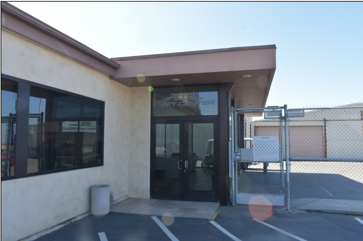
Figure 15: Continuing along the north elevation, west of Fig. 14. IS Architecture, 2019.
