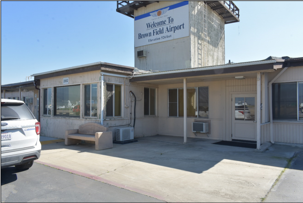
Figure 11: Central portion of the north elevation. IS Architecture, 2019.
