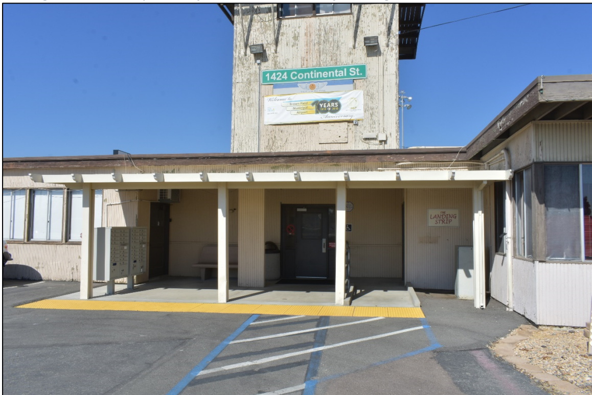
Figure 6: Main entrance at roughly the center of the southern elevation. IS Architecture, 2019.
