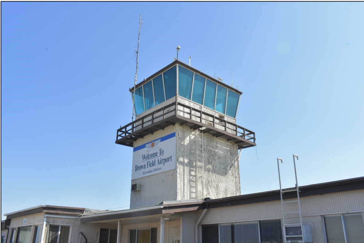
Figure 12: North and west sides of the control tower. IS Architecture, 2019.
